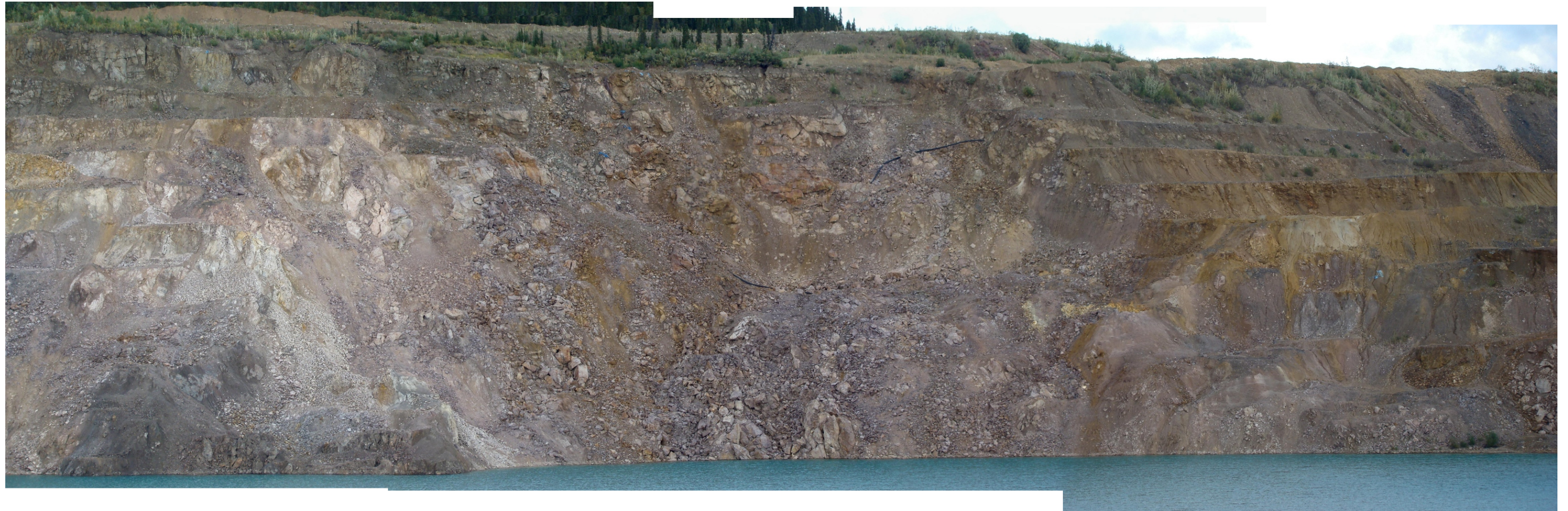
Photograph 12 : South instability zone. (August 2009).
