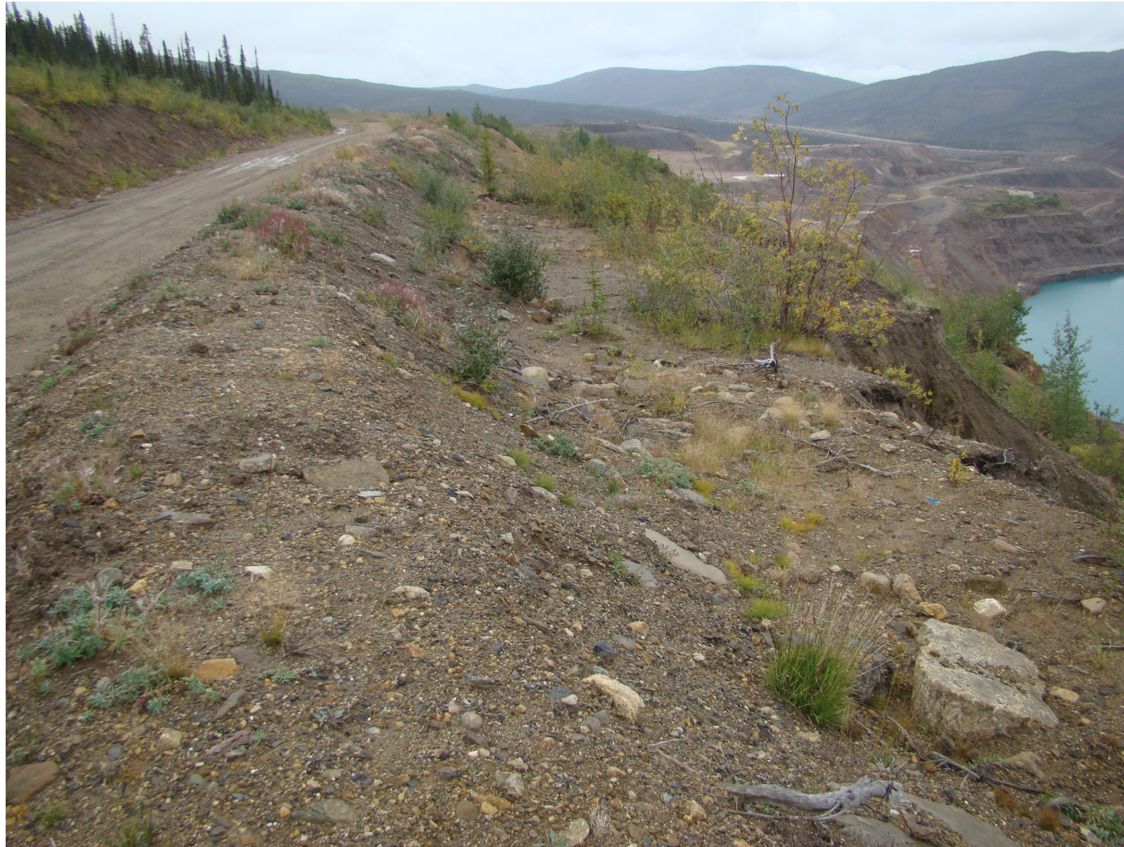
Photograph 9 : North instability zone. Minimum distance area near reference bar 15353 (August 2009).
