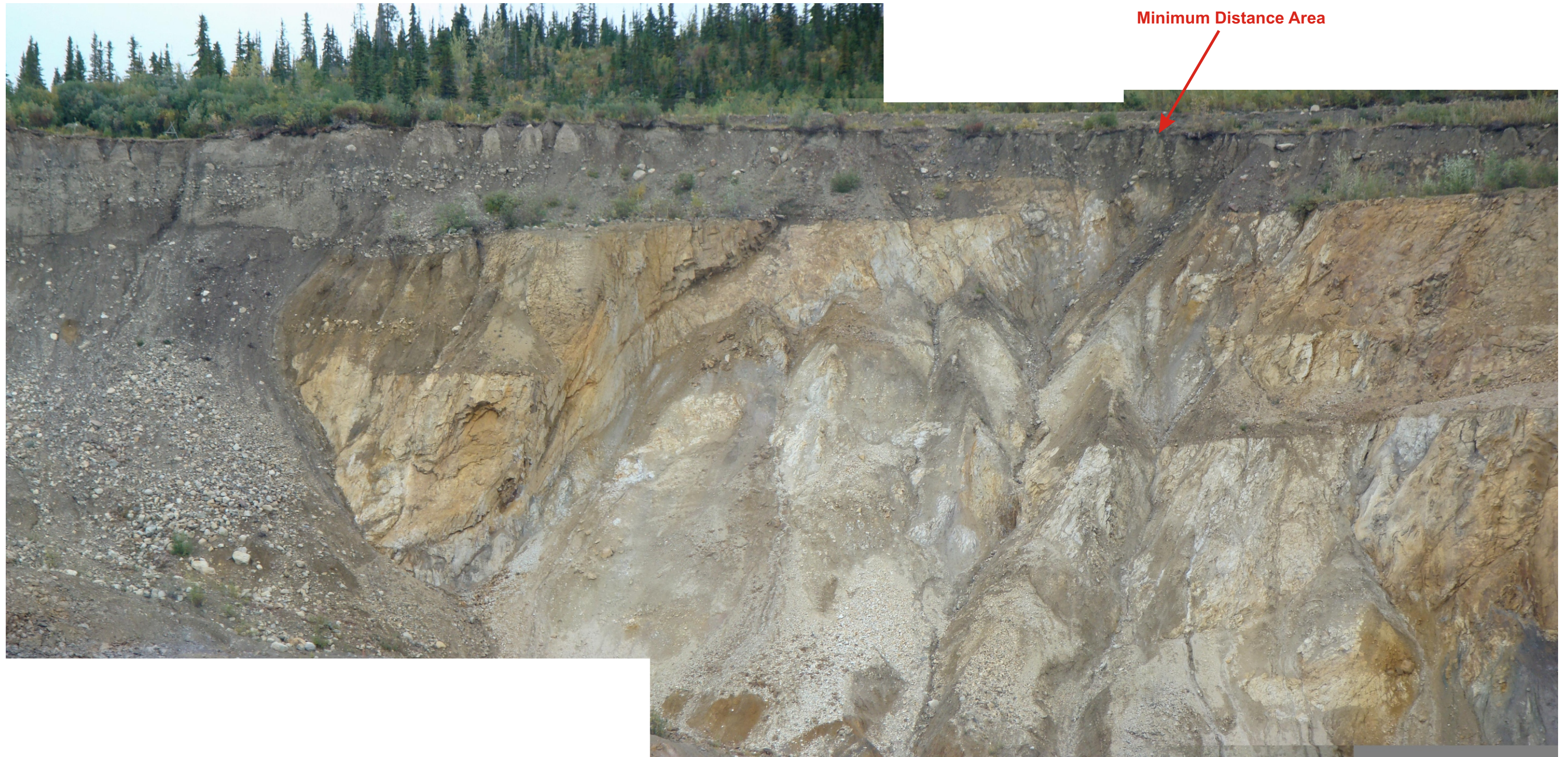
Photograph #4 : North instability zone. View of the crest of the pit wall (August 2009).
