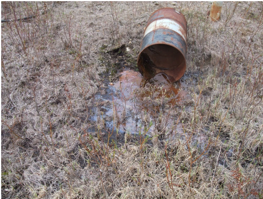
Photo 7: Seepage noted in approximately the centre of downstream face of seepage collection dam (barrel was used as a marker) June 1/12.
