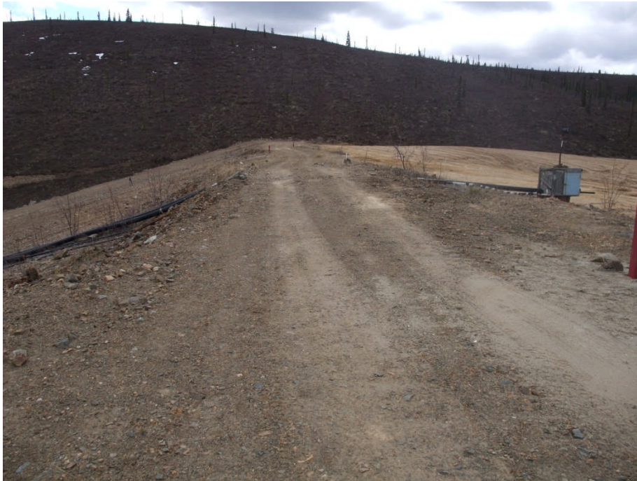
Photo 5: View to the south along crest of tailings dam (June 1/12)
