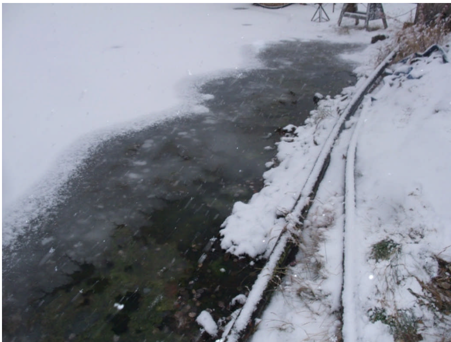
Photo 8: Seepage observed from base of sand terrace at north slope of seepage collection pond on October 1/12.
