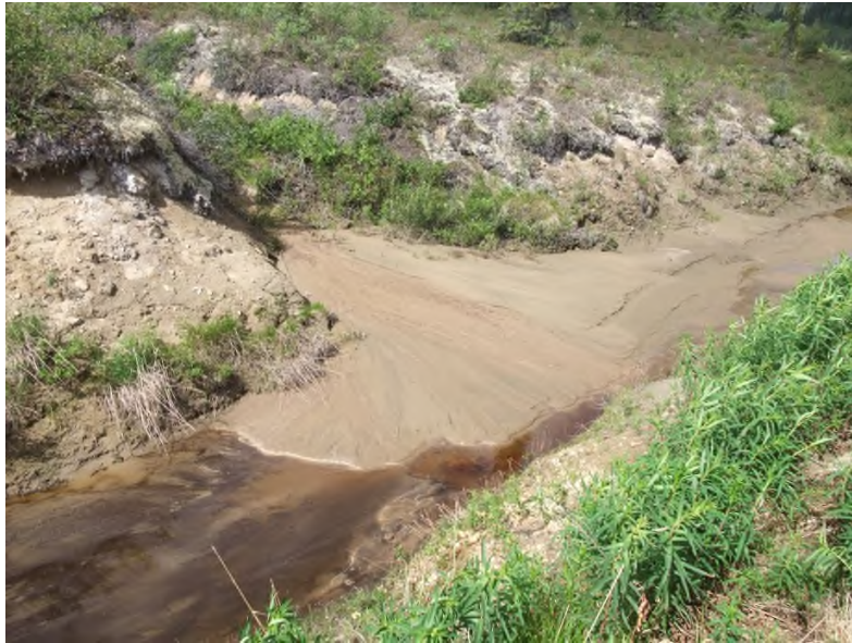
Photo 3: Sand deposits in channel bottom upstream of Dome Creek intersection (June 21/13)
