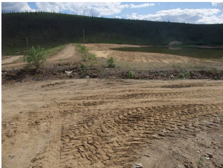
Photo 5: View to the south along crest of tailings dam (June 21/13)
