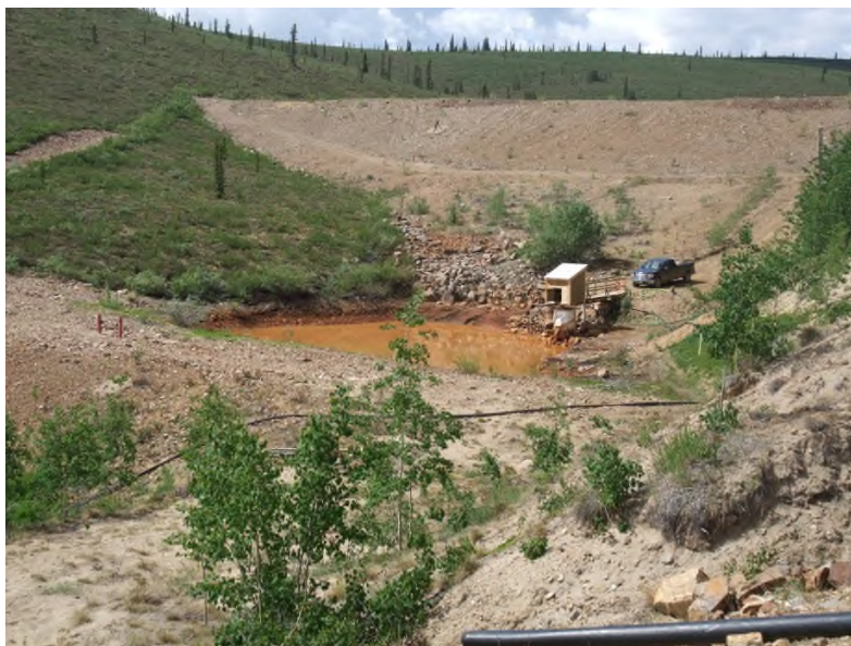
Photo 6: View of Seepage Collection Pond – water level pumped down (June 21/13).
