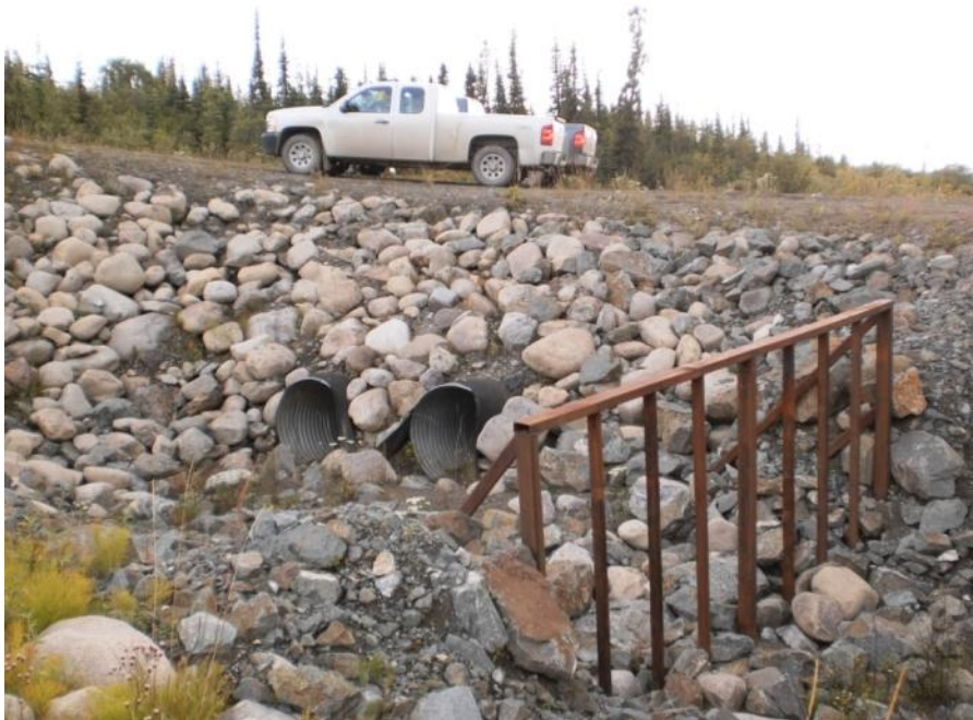
Photo 76 Vangorda Flume emergency spillway intake culverts (August 23, 2011)
