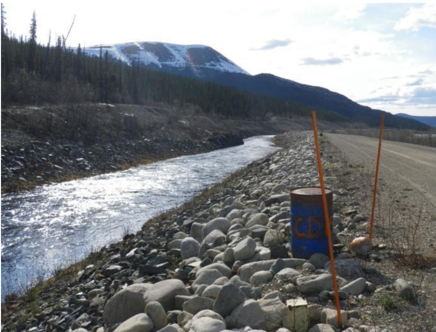
Photo 18 Channel downstream of fuse plug (May 29, 2012)
