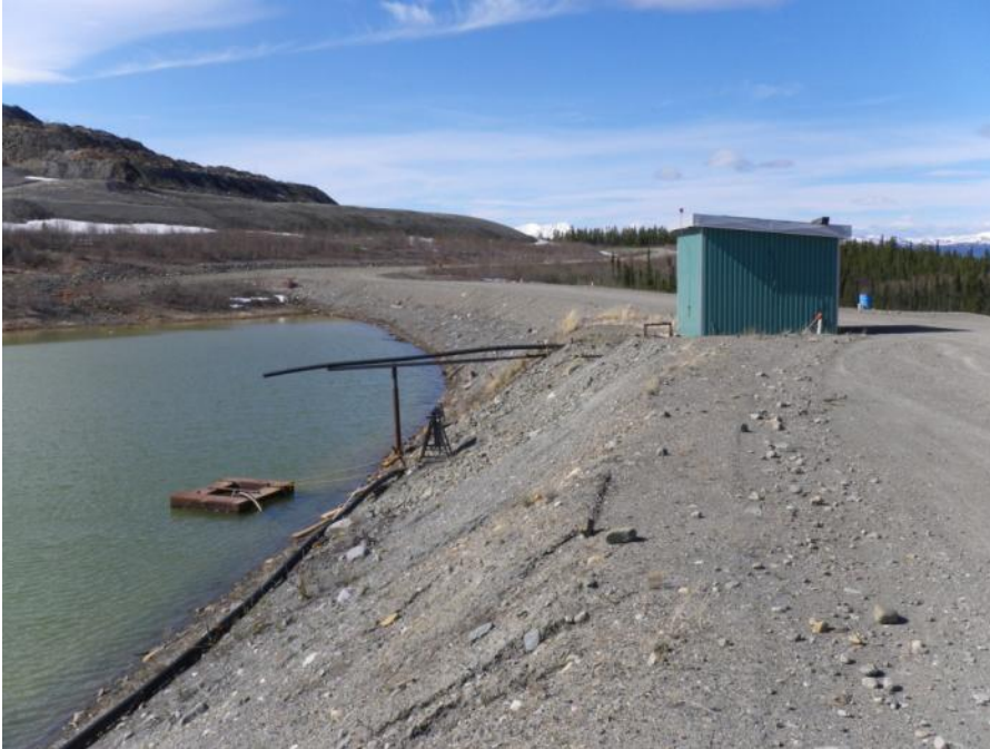
Photo 81 Little Creek Dam crest, upstream slope and Vangorda Dump seepage collection pond (May 30, 2012)
