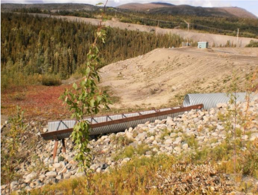
Photo 89 Crest and downstream slope/berm - emergency spillway in foreground (August 23, 2011)
