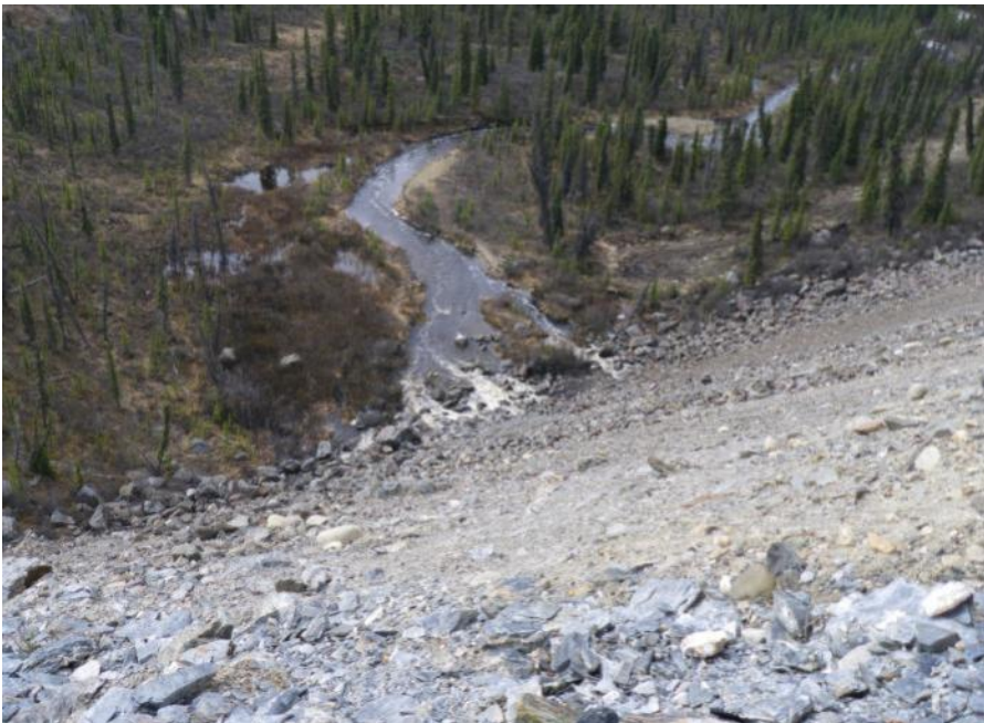
Photo 22 Downstream slope of access road at North Fork Rock Drain (May 29, 2012)
