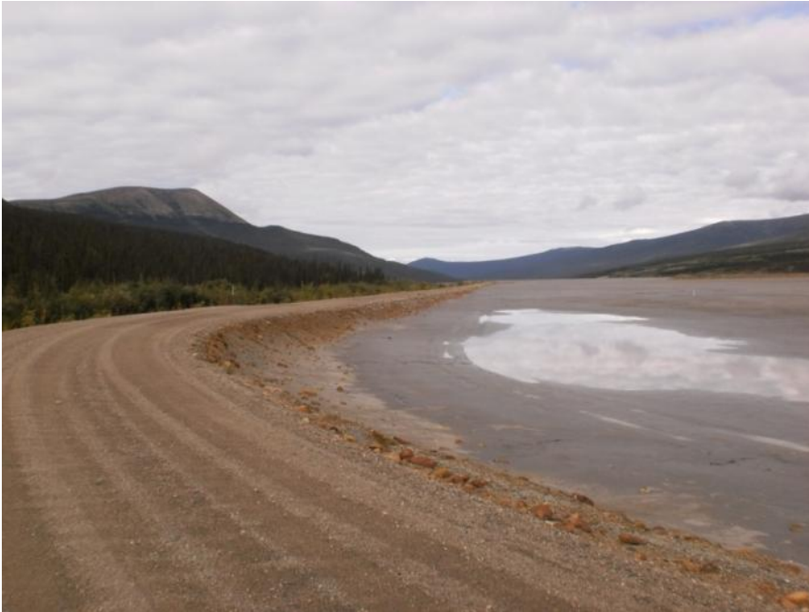
Photo 23 Southeast corner of Secondary Dam – looking northwest (August 23, 2011)
