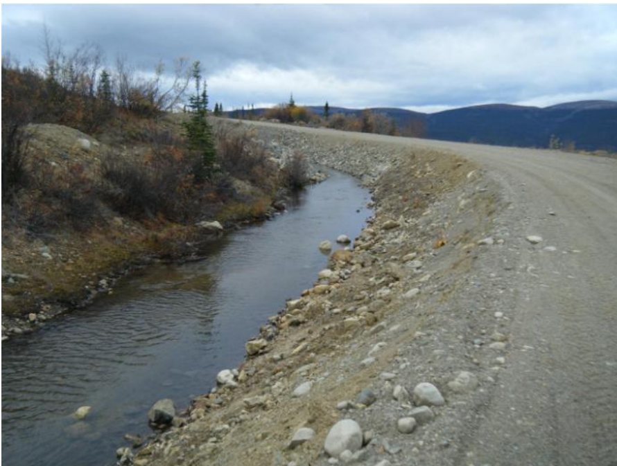
Photo 4 Faro Creek Diversion Ditch above Faro Pit, looking downstream (September 20, 2011)
