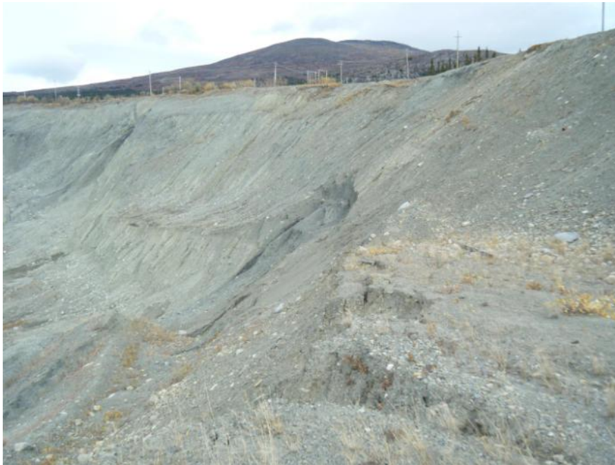
Photo 46 Grum Pit east wall - note new slump in foreground (September 20, 2011)
