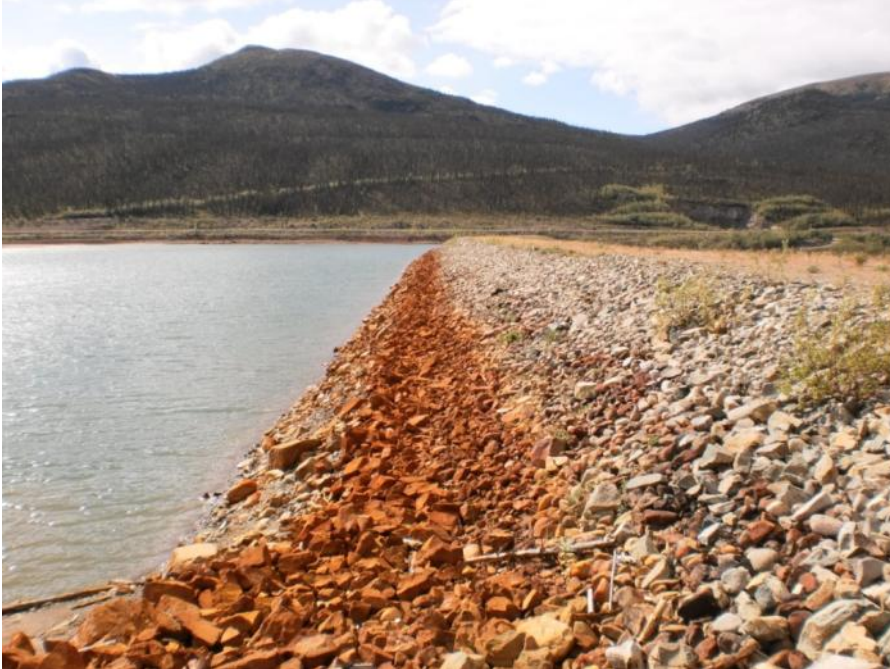
Photo 29 Upstream slope of Intermediate Dam - looking southwest (August 23, 2011)
