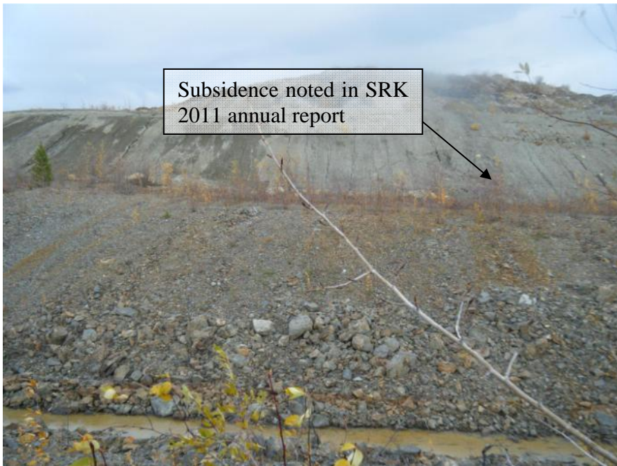
Photo 52 Vangorda Waste Dump previously noted subsidence (September 20, 2011)
