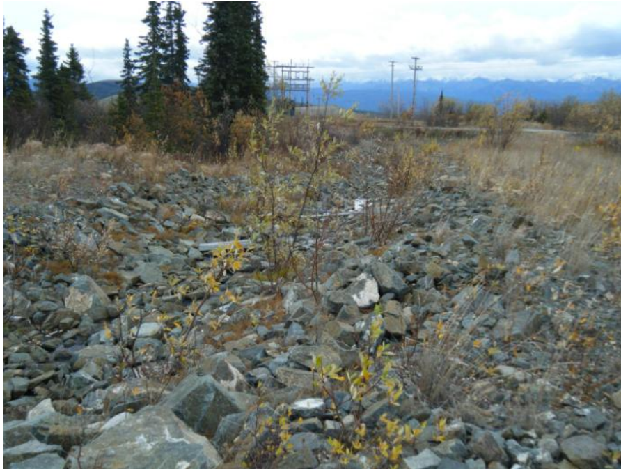
Photo 100 Grum Settling Pond spillway channel, looking downstream towards Grum Interceptor Ditch (September 20, 2011)
