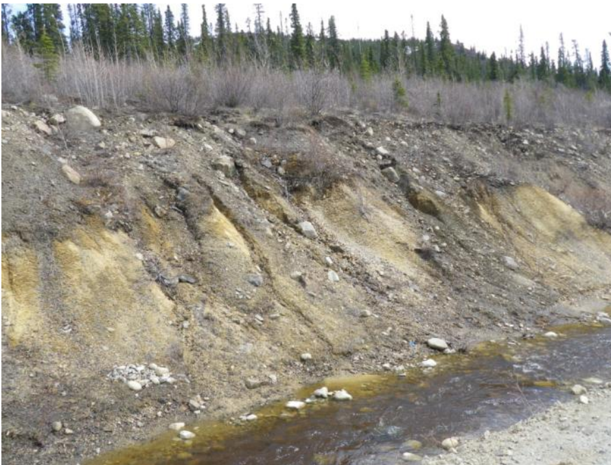
Photo 6 Slope erosions and slumps on channel bank slope (May 29, 2012).
