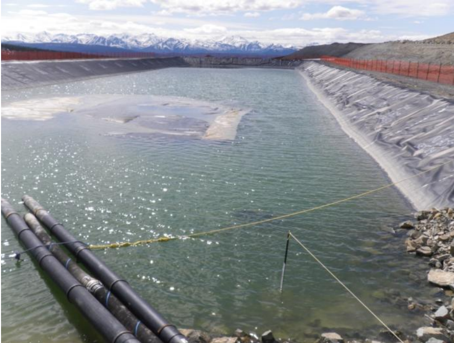
Photo 49 Grum Dump surface water storage pond (May 30, 2012)
