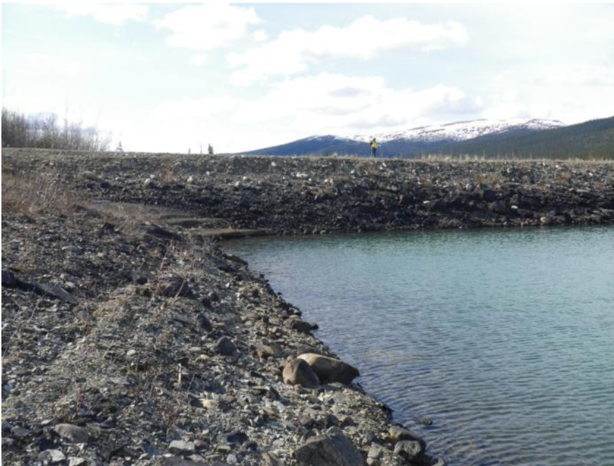
Photo 40 Canal Dyke slope upstream of Cross Valley Dam (May 29, 2012)
