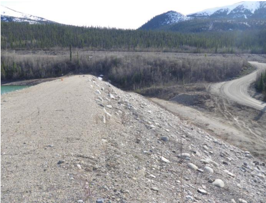
Photo 38 Dam crest and downstream slope (May 29, 2012)
