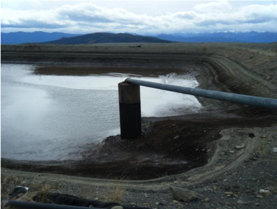
Photo 116 Grum Sludge Pond (September 20, 2011)
