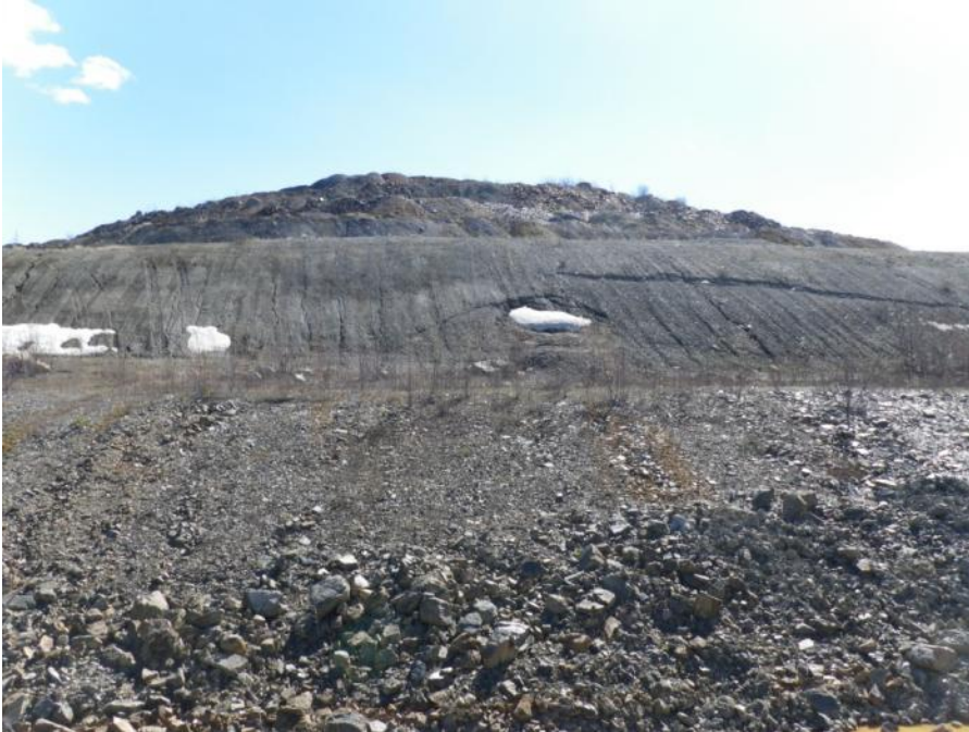
Photo 53 Dump face with previously marked slope slump (May 30, 2012)
