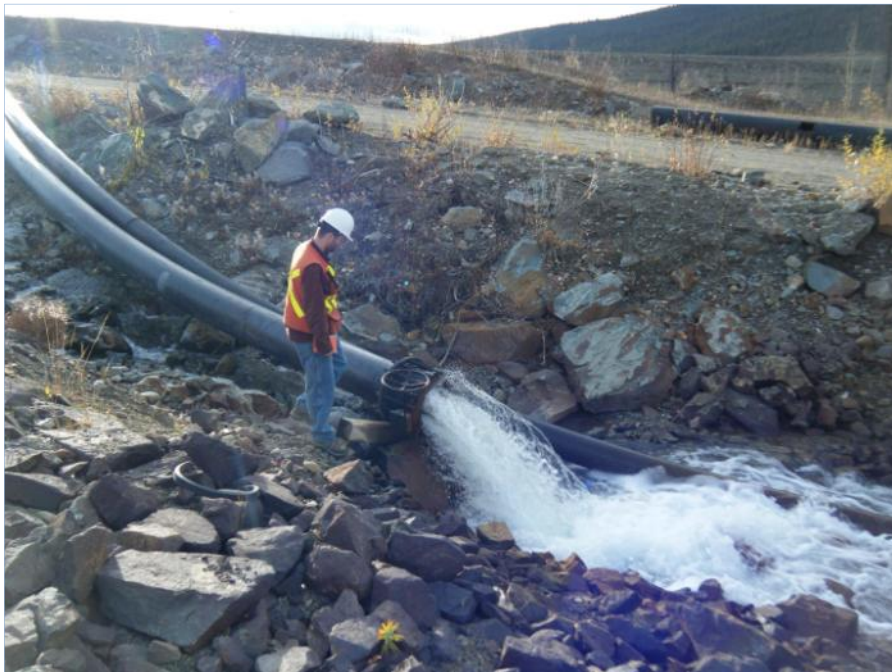
Photo 42 Cross Valley Pond siphon outlet discharge (September 20, 2011)
