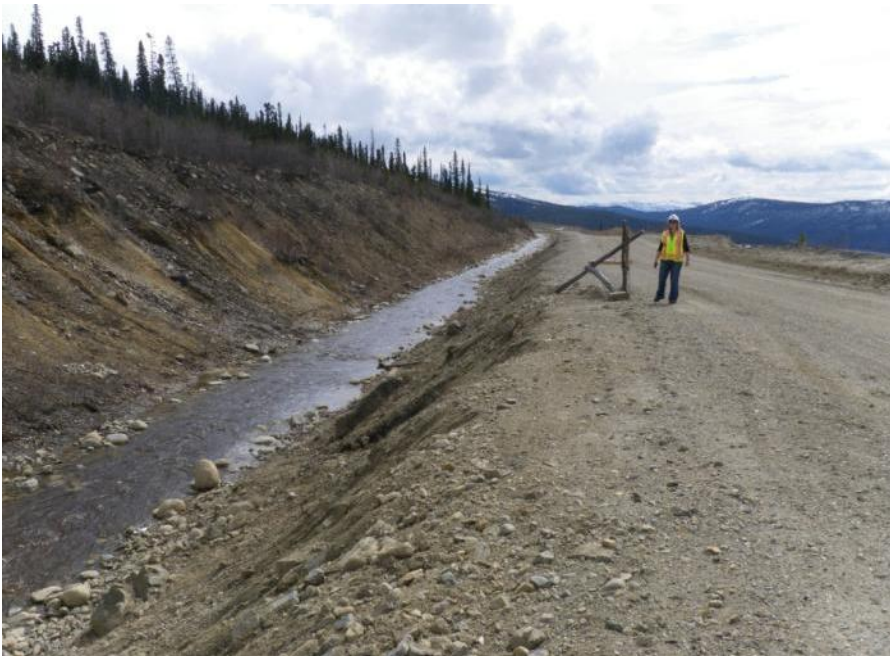
Photo 4 Diversion Channel above Faro Pit - looking downstream (May 29, 2012)
