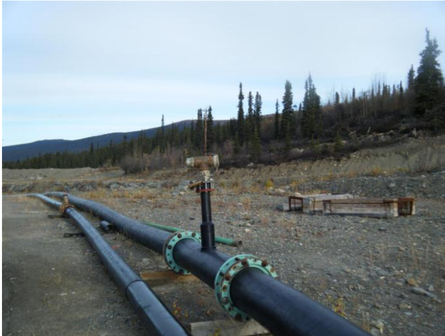
Photo 41 Cross Valley Pond siphon pipeline on spillway channel (September 21, 2011)
