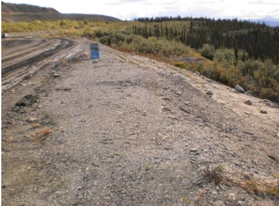
Photo 91 Crest and downstream slope/berm (August 23, 2011)
