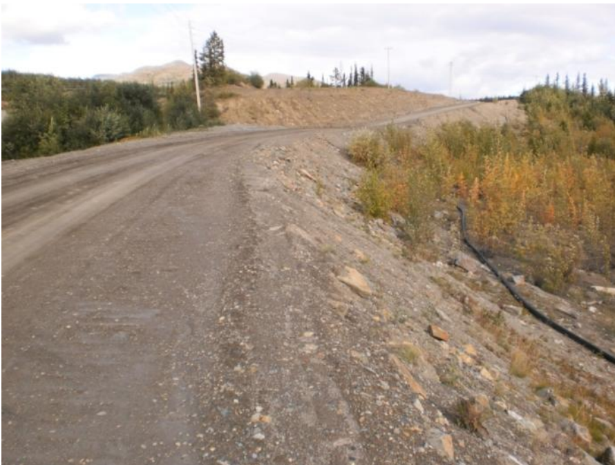
Photo 94 Dam crest and upstream slope near the north end (August 23, 2011)
