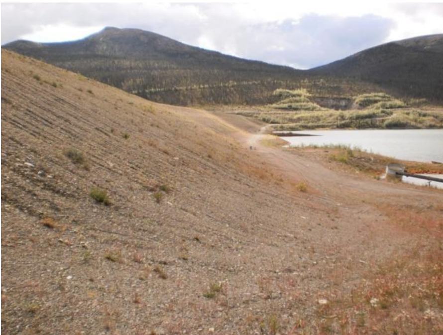
Photo 38 Northeast portion of downstream dam slope (August 23, 2011)
