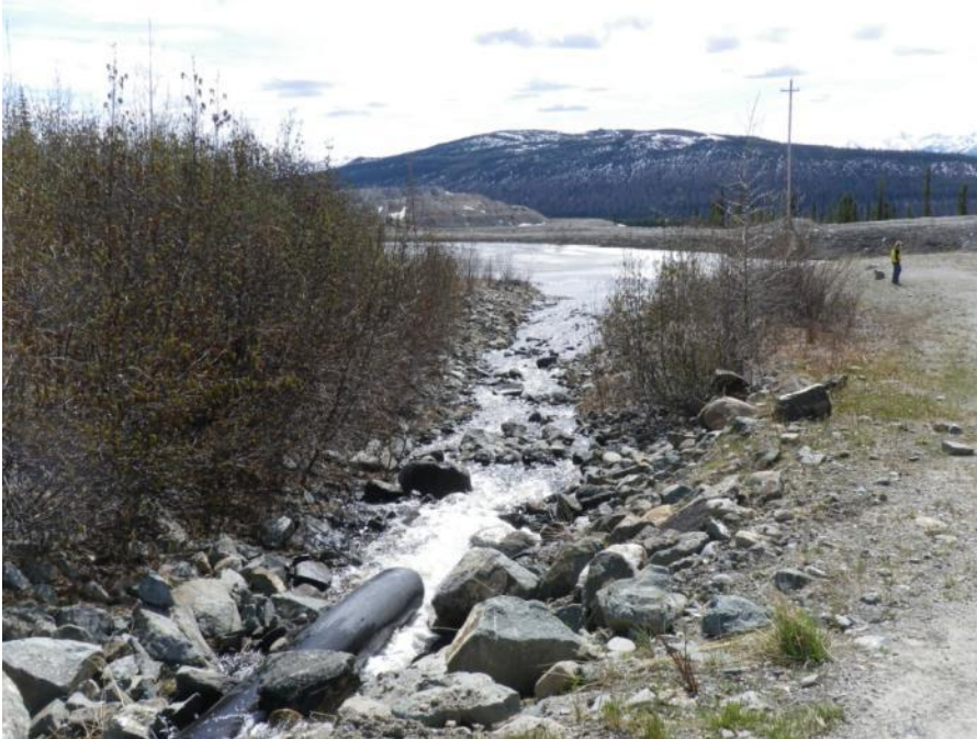
Photo 87 Flow entering Upper Sheep Pad Sediment Pond (May 30, 2012)
