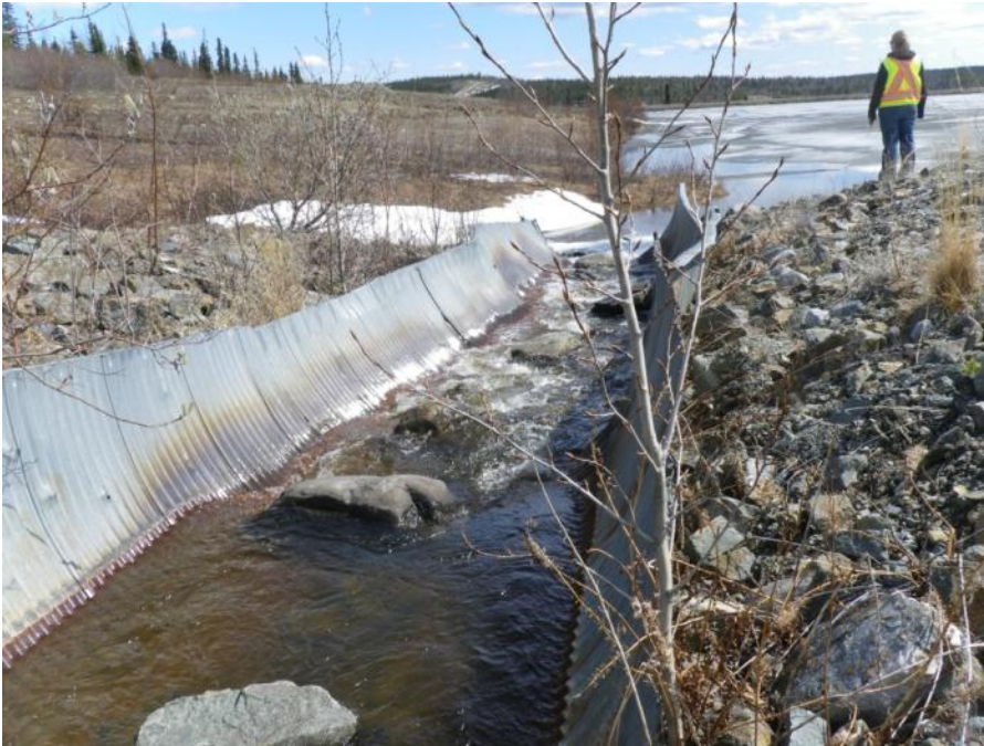
Photo 89 Flume flow from Upper to Lower Sheep Pad Pond (May 30, 2012)
