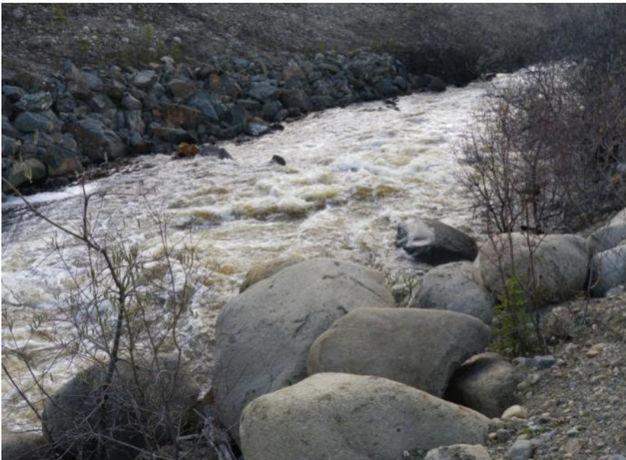
Photo 20 Diversion Channel adjacent to Cross Valley Dam looking downstream (May 29, 2012)
