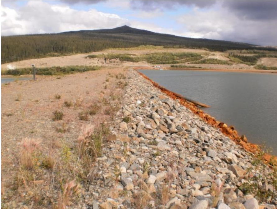
Photo 33 Southwest portion of dam crest and upstream slope (August 23, 2011)
