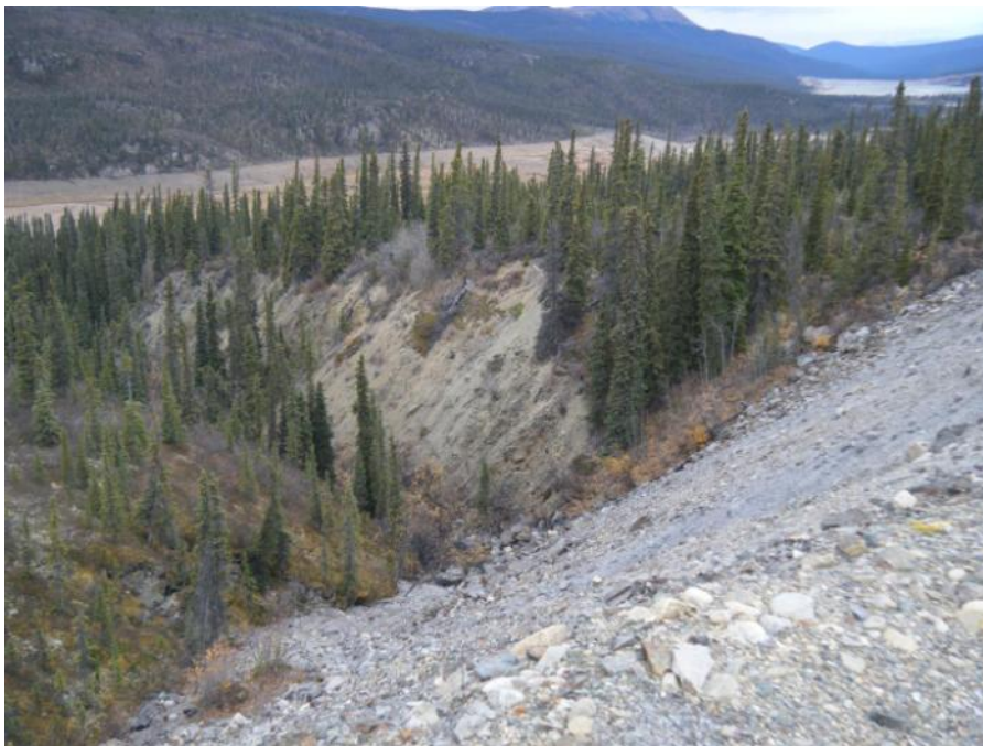
Photo 20 K8 Creek downstream outlet (September 20, 2011)
