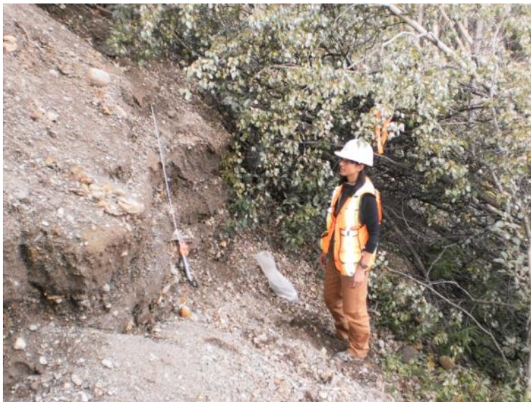
Photo 113 Downstream bank slope of esker
