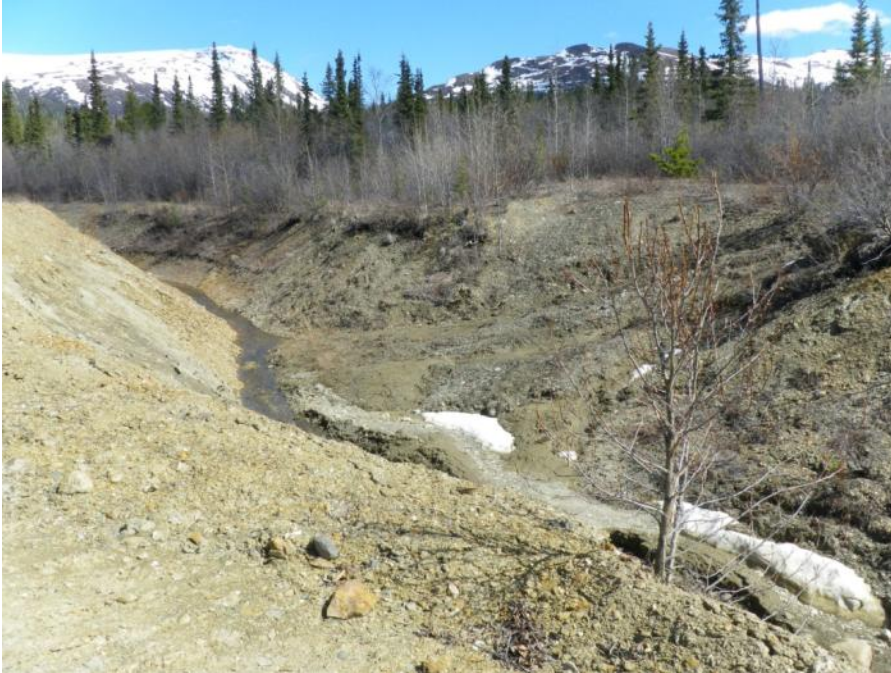
Photo 67 Ditch bank slope slump (May 30, 2012)
