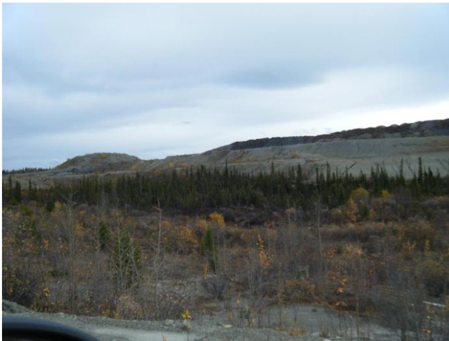
Photo 50 Vangorda Waste Dump (September 20, 2011)
