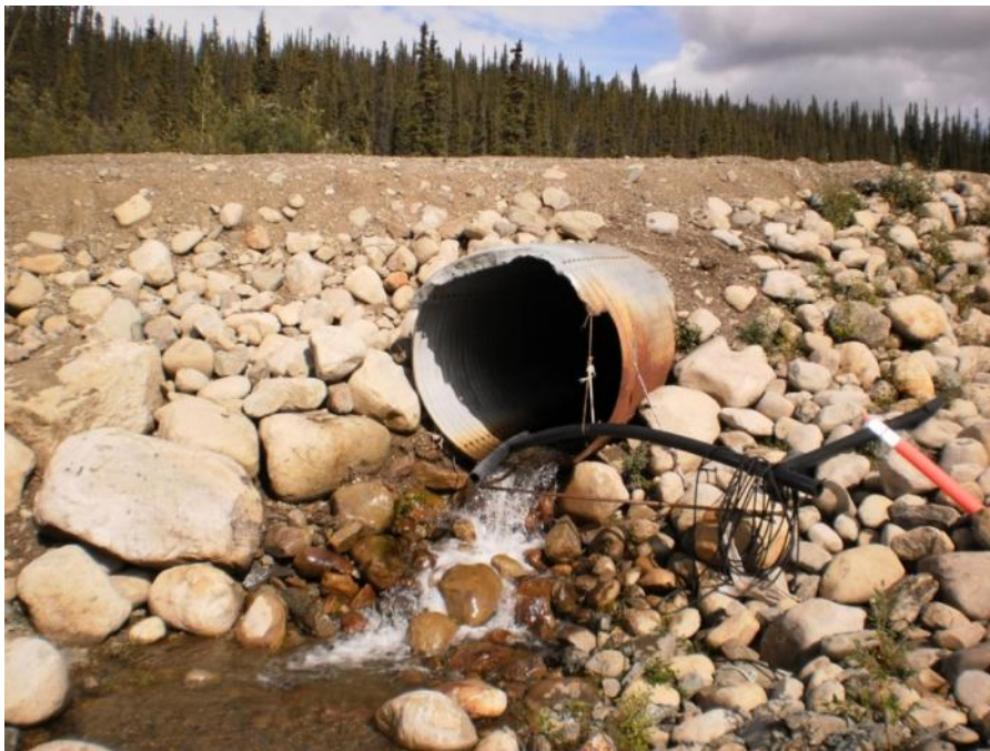
Photo 8 Culvert discharge from Interceptor Ditch adjacent to Cross Valley Pond (August 23, 2011)
