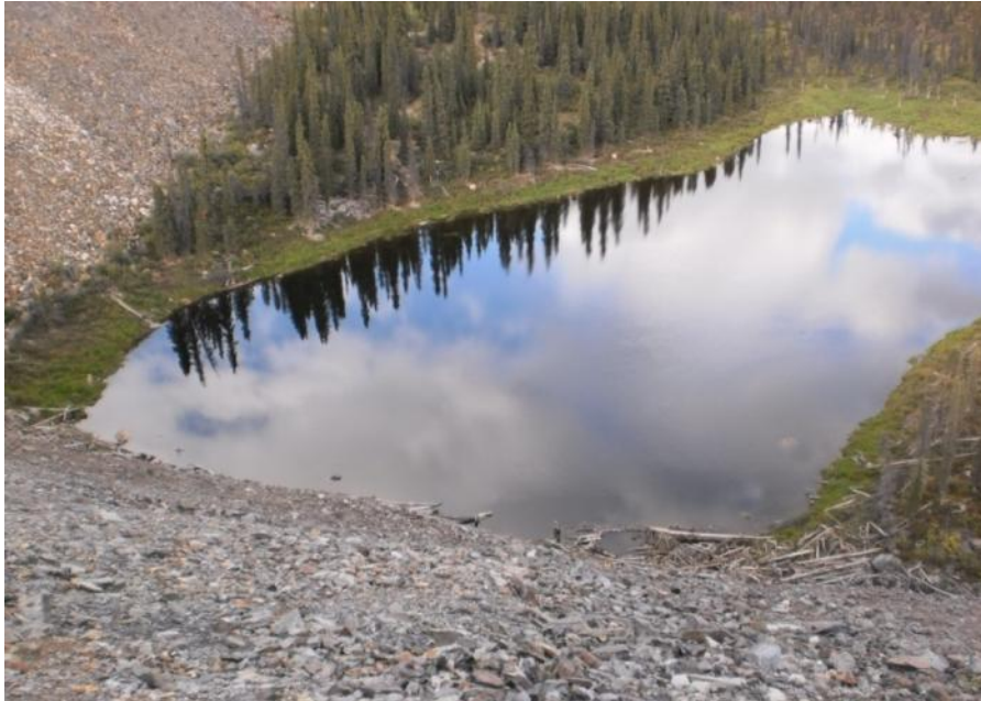
Photo 17 Wood debris on upstream slope of Access Road between Faro and Vangorda Plateau (August 23, 2011)
