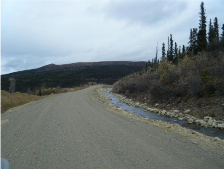
Photo 3 Faro Creek Diversion Ditch above Faro Pit, looking upstream (September 20, 2011)
