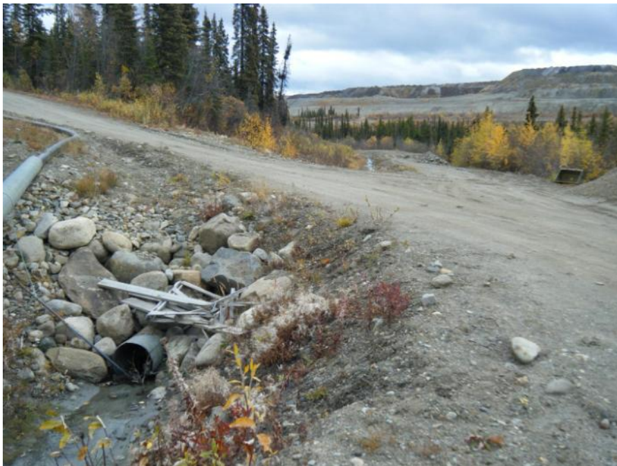
Photo 104 V-15 Diversion Ditch looking downstream towards Moose Pond (September 20, 2011)
