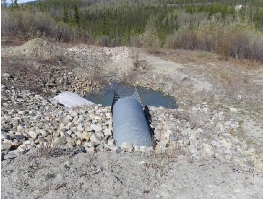
Photo 85 Culvert spillway outlet (May 30, 2012)
