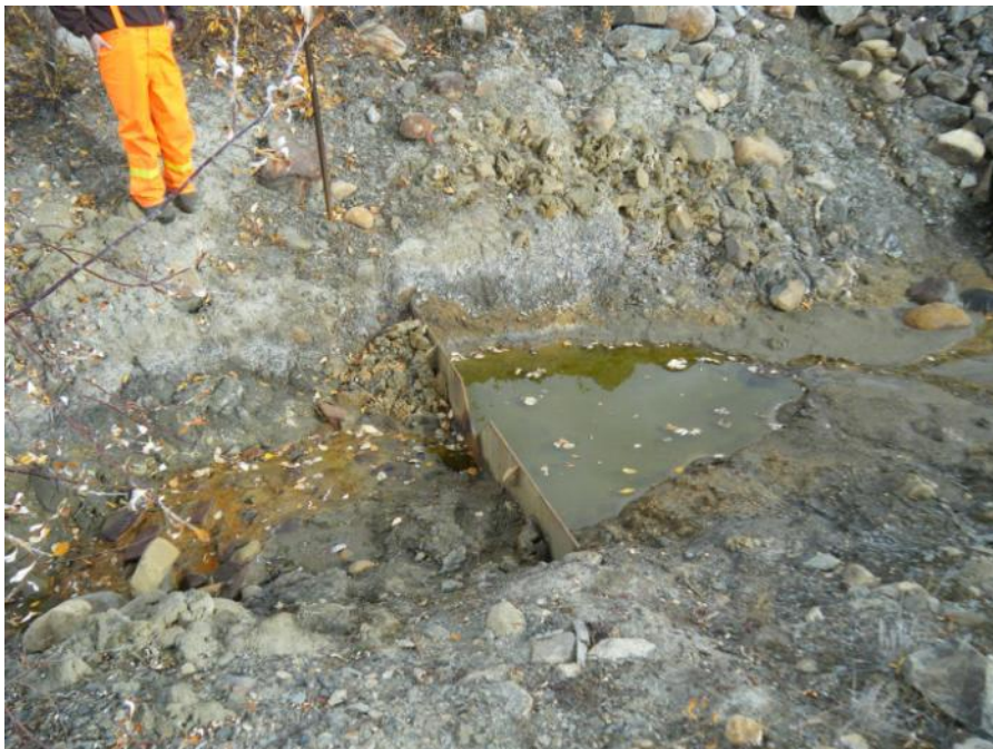
Photo 64 Vangorda Waste Dump Drain No. 6. weir (September 20, 2011)
