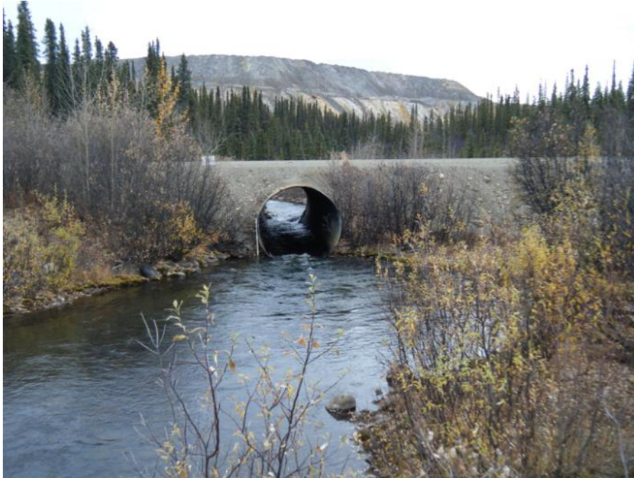
Photo 11 Rose Creek North Fork culvert under main road (September 21, 2011)
