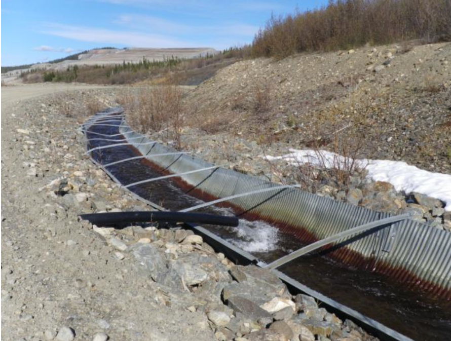
Photo 71 Inflow to Flume Diversion by pumping from intercepted runoff collected below access road (May 30, 2012)
