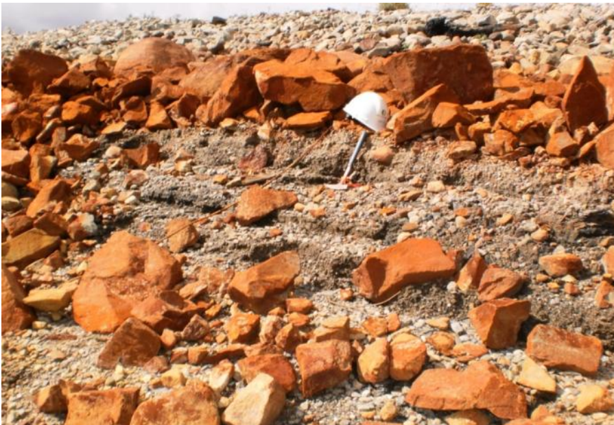
Photo 30 Wave erosion zone on upstream slope marked by hard hat and hammer (August 23, 2011)
