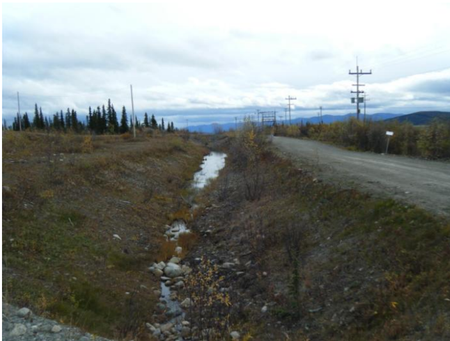
Photo 68 Grum Interceptor Ditch near Grum Water Treatment Plant (WTP), looking downstream (September 20, 2011)
