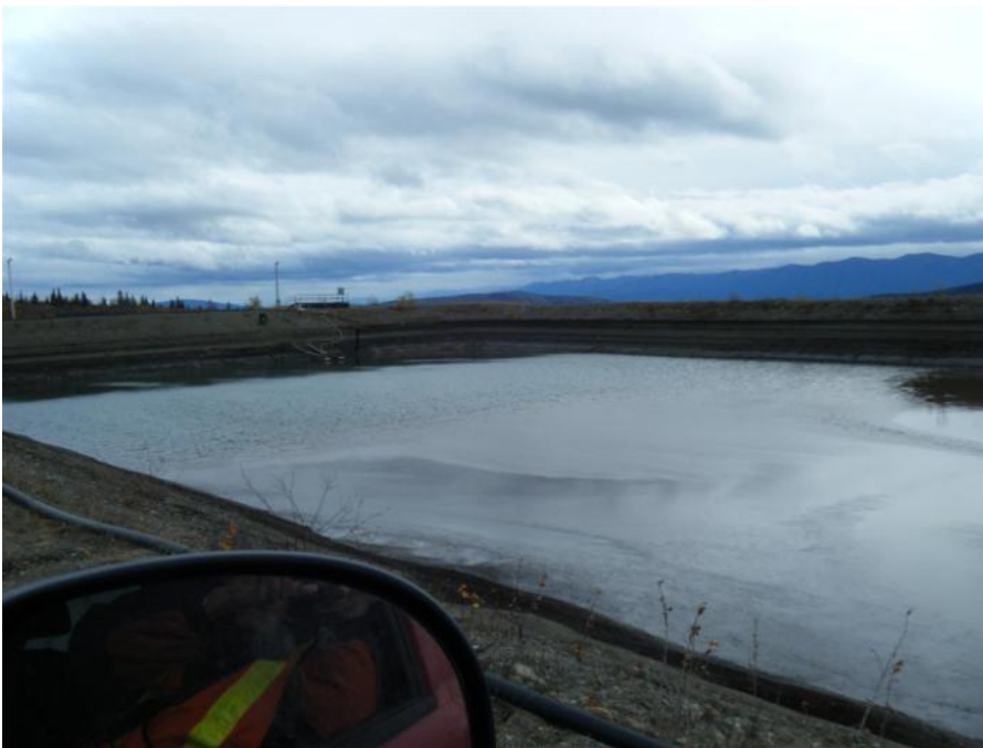
Photo 117 Grum Sludge Pond (September 20, 2011)
