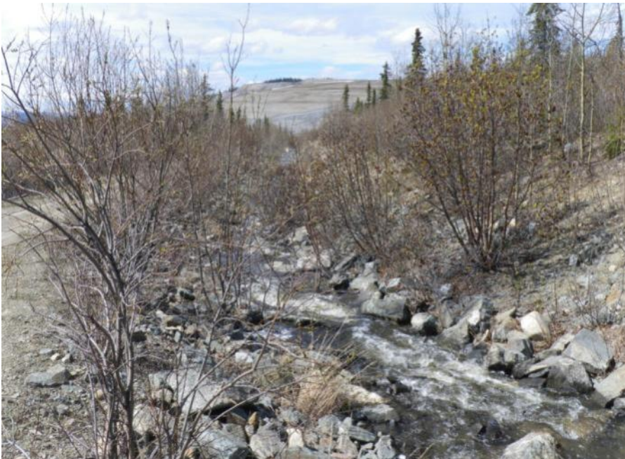
Photo 62 Interceptor Ditch flowing towards Sheep Pad Sediment Ponds (May 30, 2012).
