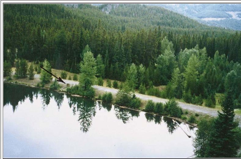
Figure 17 – Excess growth, broken log boom
