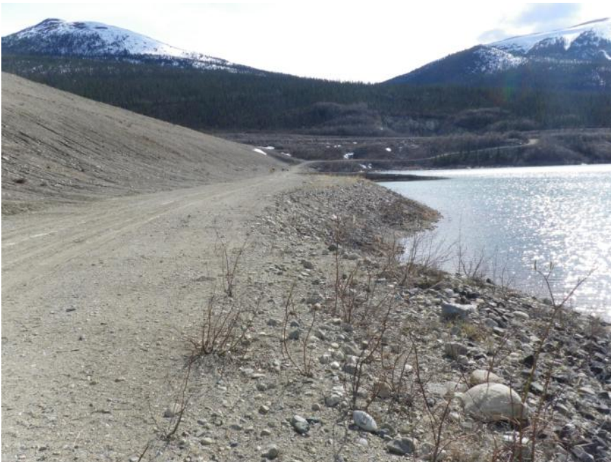
Photo 36 Downstream slope of downstream berm (May 29, 2012)
