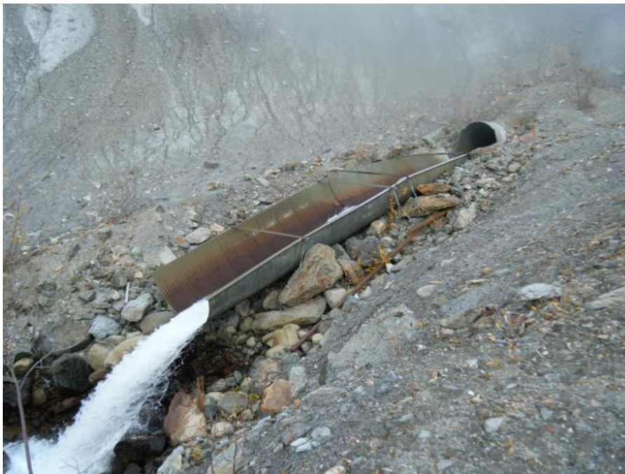
Photo 86 Vangorda Creek Diversion outfall at Vangorda Creek downstream of drop box (September 20, 2011)
