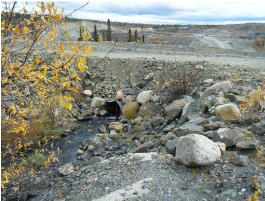
Photo 96 Culvert downstream of Sheep Pad Sediments Ponds weir
