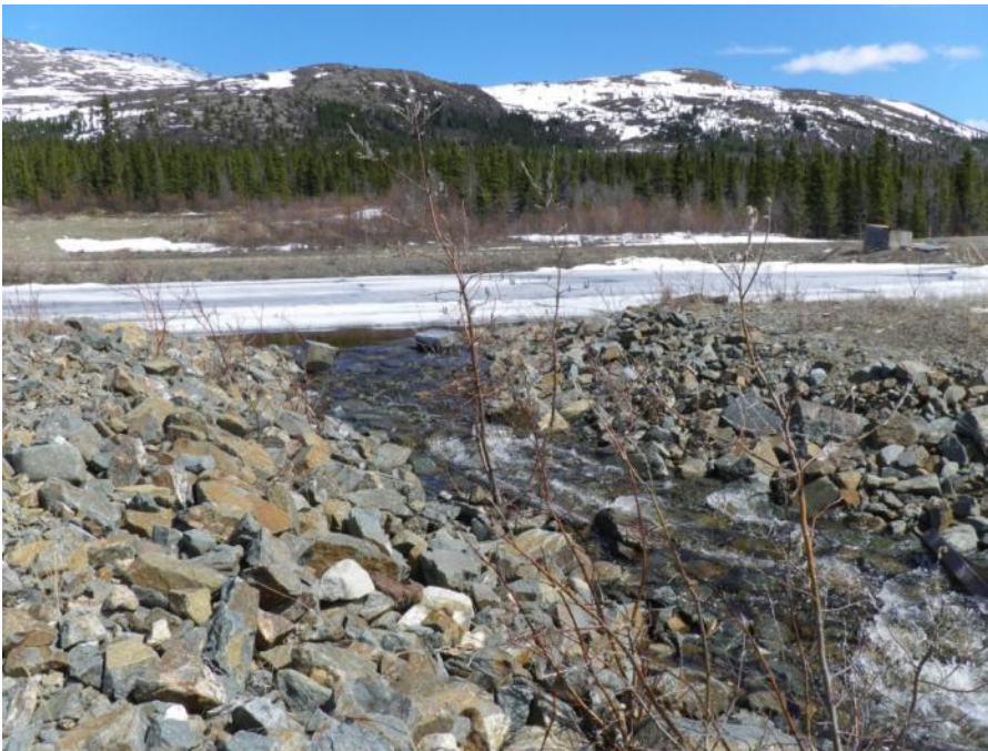
Photo 92 Grum Settling Pond and flow through spillway channel (May 30, 2012)
