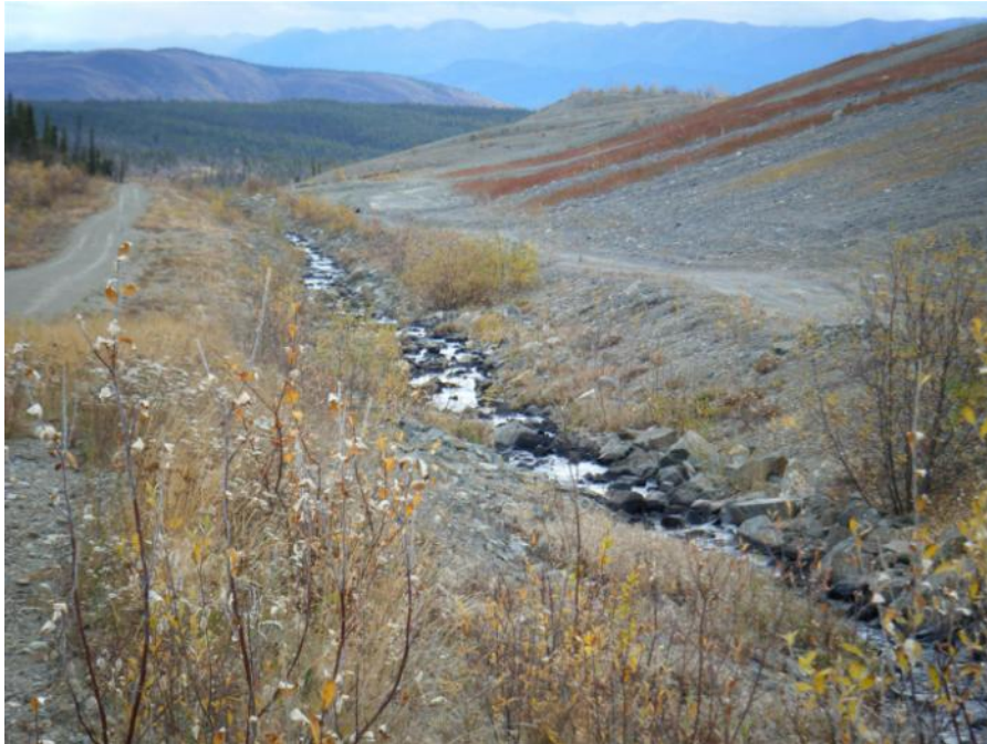
Photo 69 Grum Interceptor Ditch along toe of Overburden Dump. Note vegetation test plots on dump face
