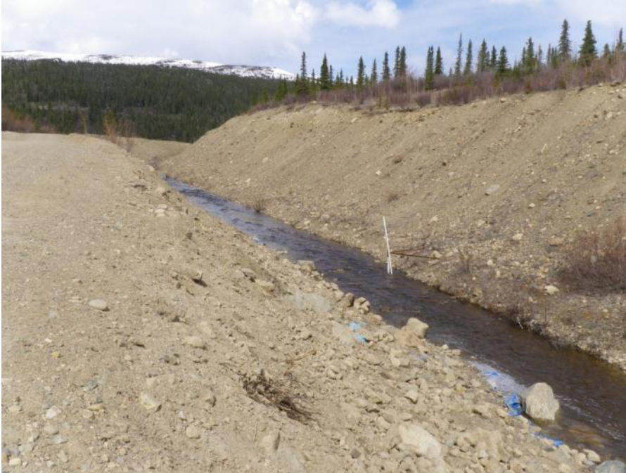
Photo 3 Faro Creek Diversion Channel above Faro Pit - looking upstream (May 29, 2012)
