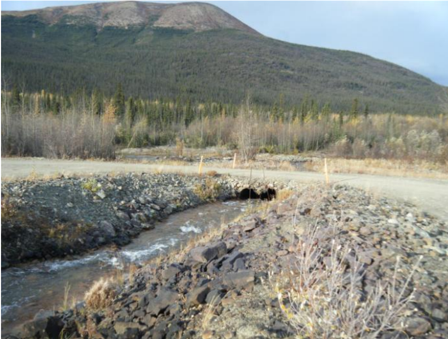
Photo 9 Interceptor Ditch culverts across access road below Cross Valley Dam (September 20, 2011)
