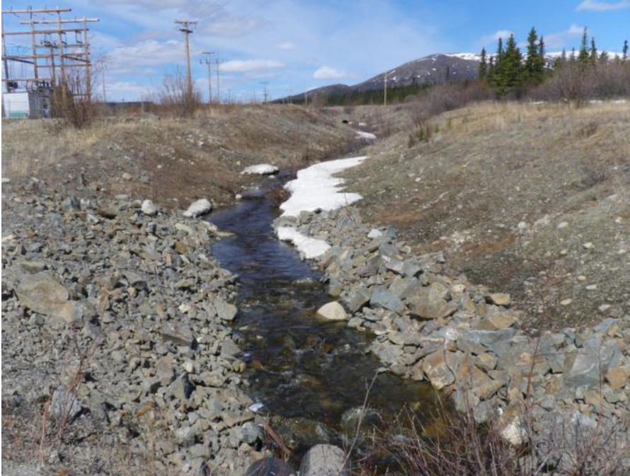
Photo 59 Grum Pit Interceptor Ditch in vicinity of power substation(May 30, 2012)
