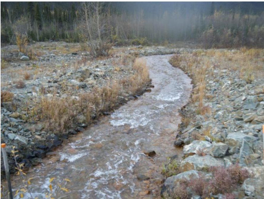
Photo 10 Interceptor Ditch below Cross Valley Dam, looking downstream (September 20, 2011)
