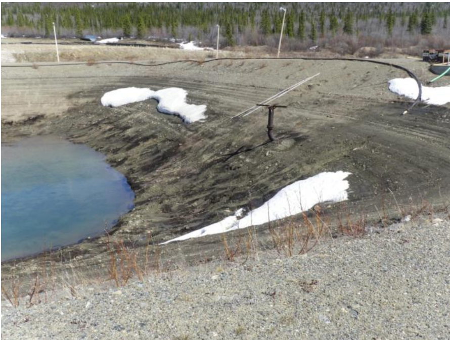
Photo 102 Sludge Pond (May 30, 2012)
