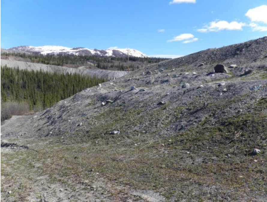
Photo 83 Downstream dam and berm slope (May 30, 2012)
