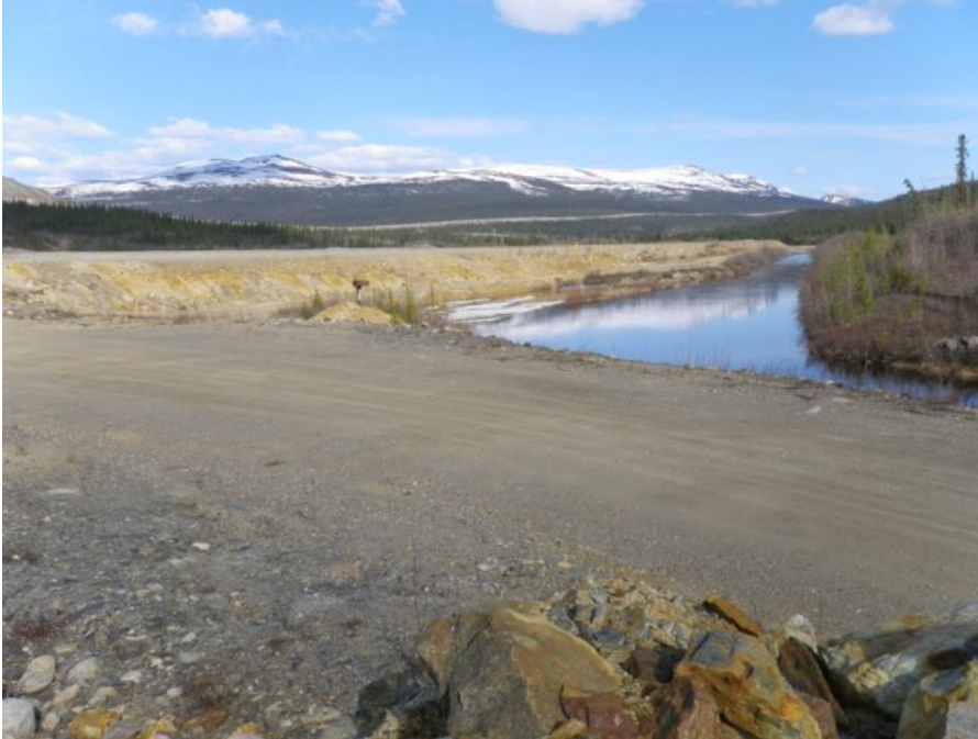
Photo 17 Rose Creek Diversion Channel upstream of fuse plug (May 29, 2012)
