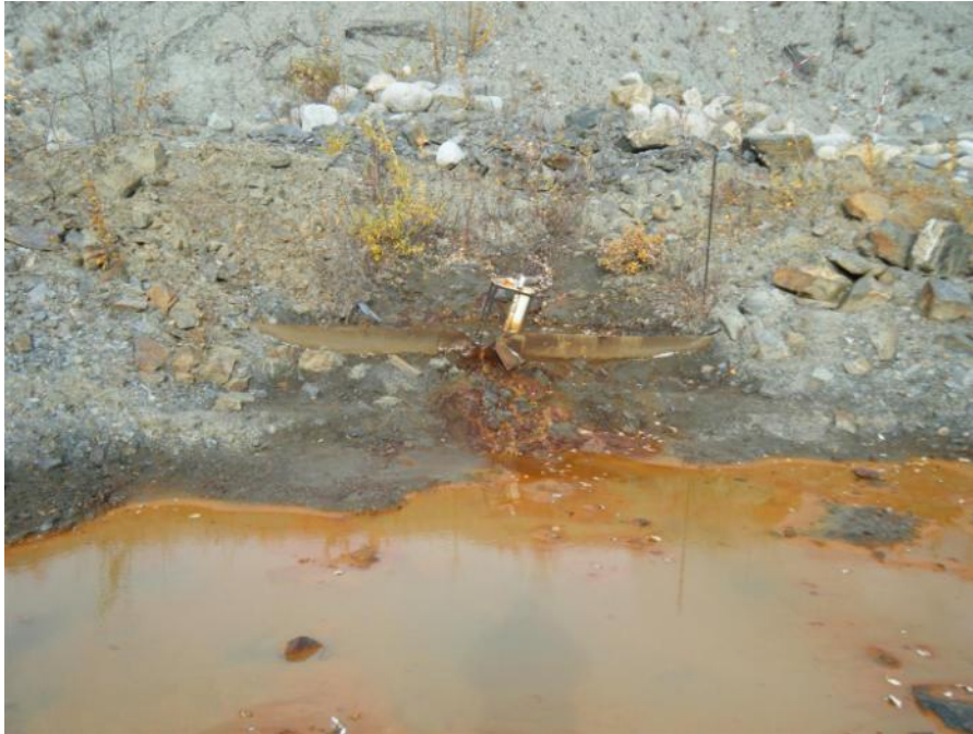
Photo 57 Vangorda Waste Dump Drain No. 3 weir (September 20, 2011)
