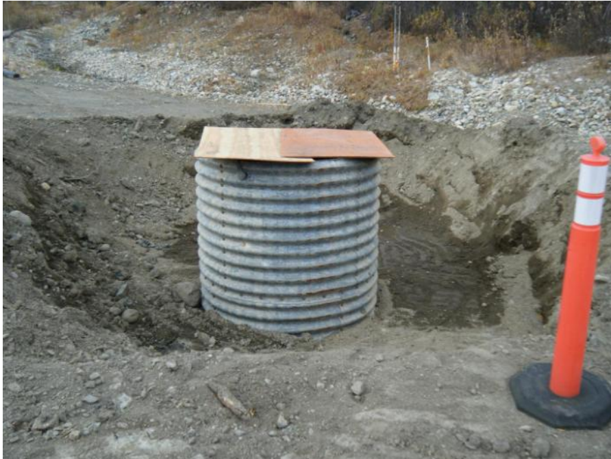
Photo 105 V-15 Pump Sump under construction (September 20, 2011)
