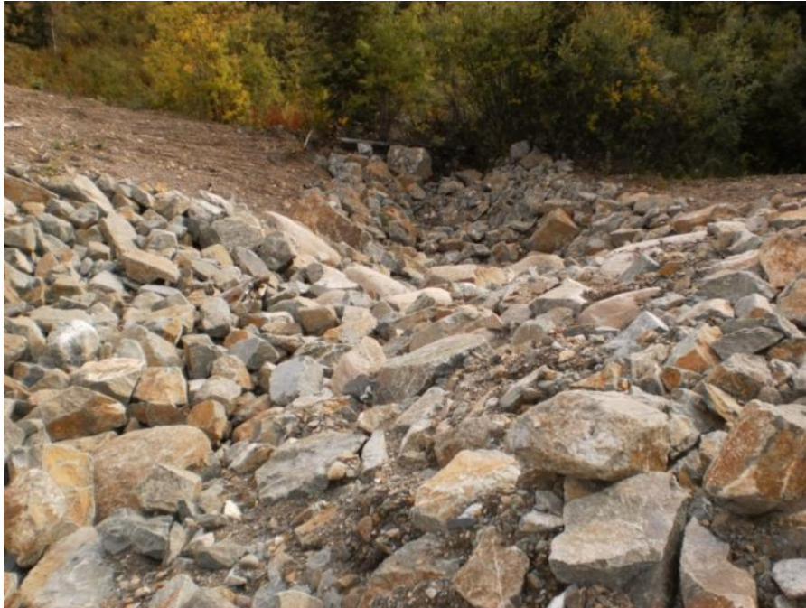
Photo 109 Downstream portion of V-15 Ditch discharge channel
