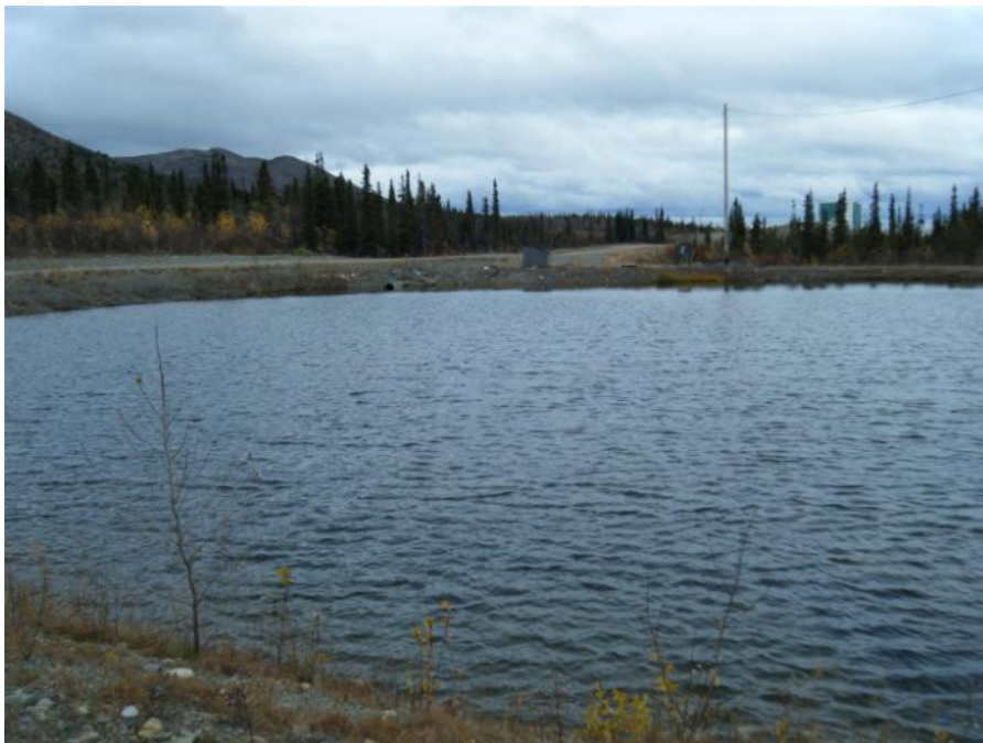
Photo 99 Grum Settling Pond (September 20, 2011)
