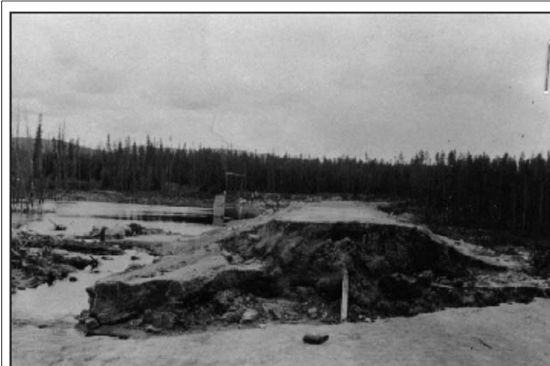
Figure 6 – Ellis Creek Dam Failure (near Penticton) 1941
