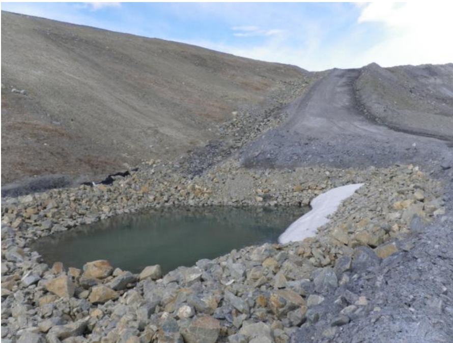
Photo 50 Grum Dump side slope, water retention pond on bench and access ramp (May 30, 2012).
