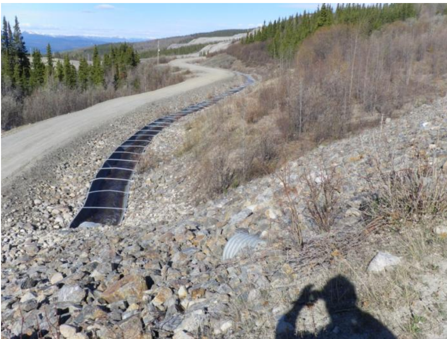
Photo 70 Culvert flow into Vangorda Flume Diversion (May 30, 2012)
