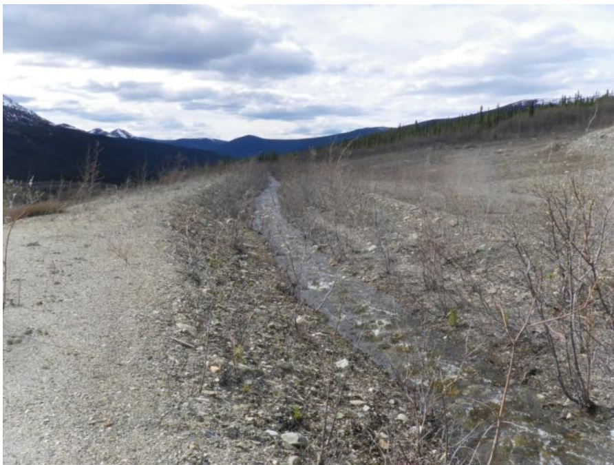
Photo 12 Middle reach of Interceptor Ditch (May 30, 2012)
