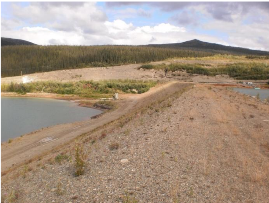
Photo 32 Northeast portion of dam crest and upstream slope (August 23, 2011)
