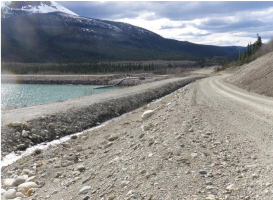
Photo 16 Interceptor Ditch lower reach adjacent to Cross Valley Pond (May 30, 2012)
