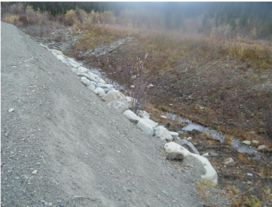
Photo 66 Grum Interceptor Ditch (September 20, 2011)
