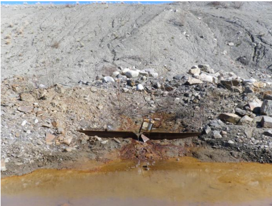
Photo 52 Vangorda Waste Rock Dump drain no. 3 (May 30, 2012)
