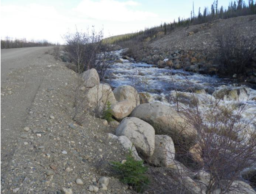
Photo 19 Diversion Channel adjacent to Cross Valley Dam looking upstream (May 29, 2012)
