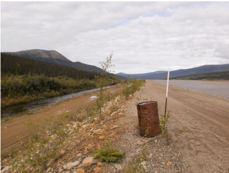
Photo 24 Secondary Tailings Dam - Rose Creek Diversion Channel on left and tailings beach on right (August 23, 2011)
