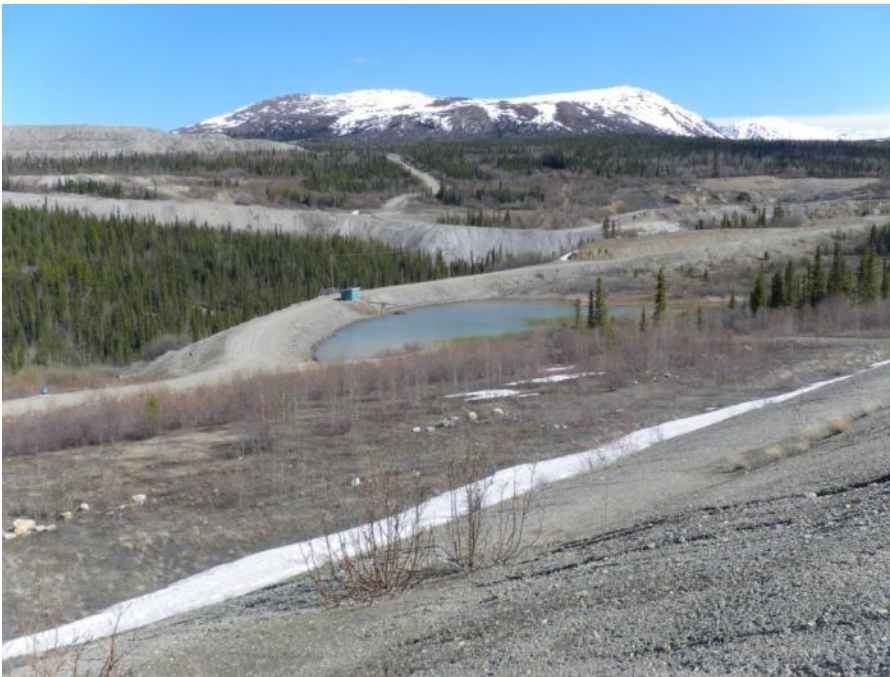
Photo 56 Toe of dump slope in area above Little Creek Dam (May 30, 2012)
