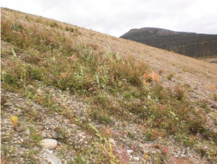
Photo 37 Less rill erosion over vegetated portion of downstream slope (August 23, 2011)
