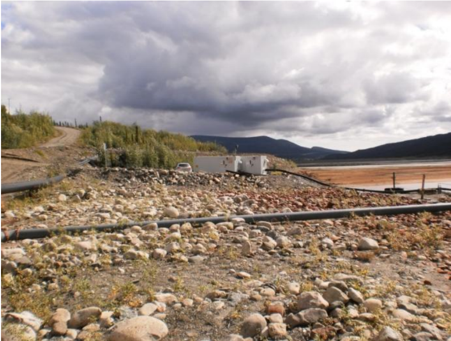
Photo 27 Upstream spillway approach channel at northeast abutment of Intermediate Dam (August 23, 2011)
