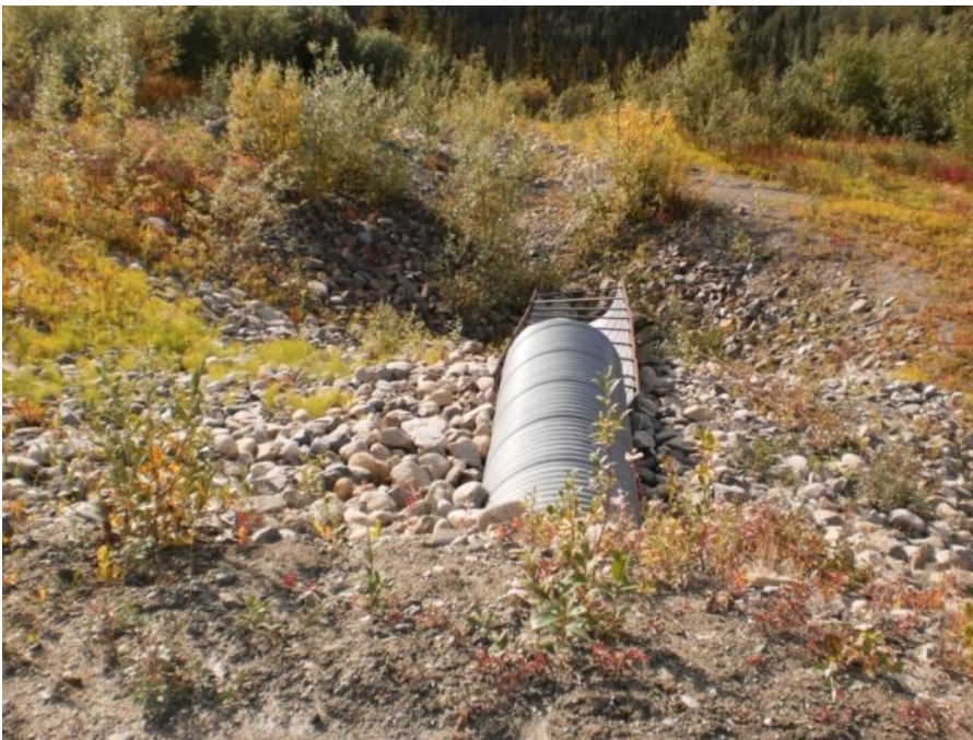
Photo 88 Culvert emergency spillway at left (south) abutment (August 23, 2011)
