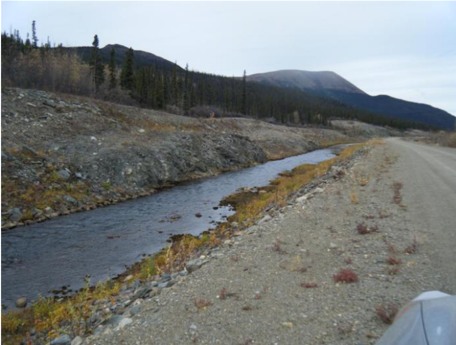
Photo 13 Rose Creek Diversion Channel downstream of Fuse Plug (September 21, 2011)
