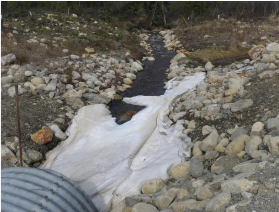
Photo 14 Entrance to culvert leading to lower reach of Interceptor Ditch (May 30, 2012).
