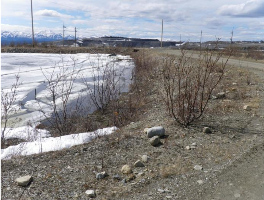
Photo 91 Grum Settling Pond (May 30, 2012)
