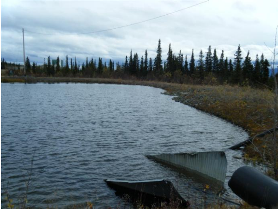
Photo 98 Grum Settling Pond (September 20, 2011)
