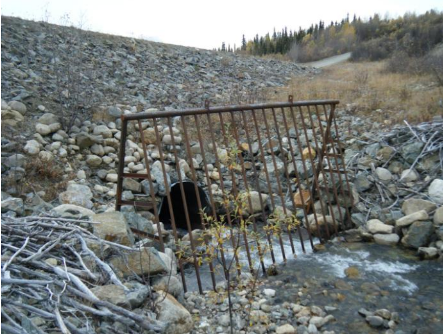
Photo 77 Vangorda Flume intake culvert (September 20, 2011)
