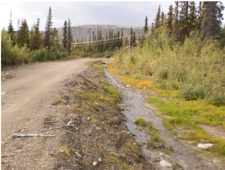
Photo 106 V-15 Diversion Ditch (August 23, 2011)
