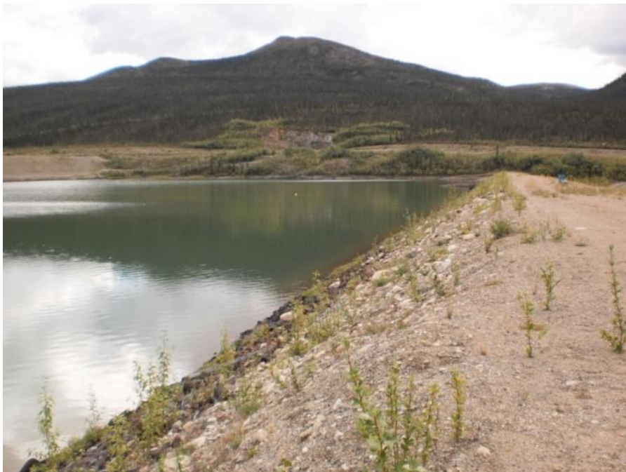
Photo 40 Crest and upstream slope of northeast portion of dam (August 23, 2011)
