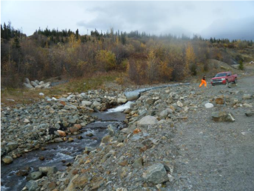
Photo 83 Downstream end of Vangorda Flume above plunge pool (September 20, 2011)
