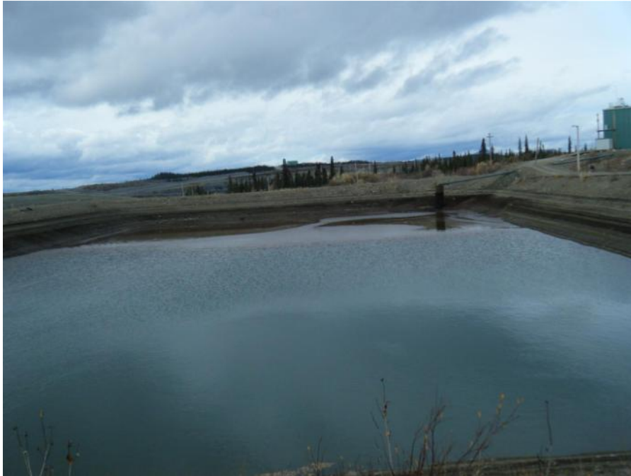
Photo 118 Grum Sludge Pond (September 20, 2011)
