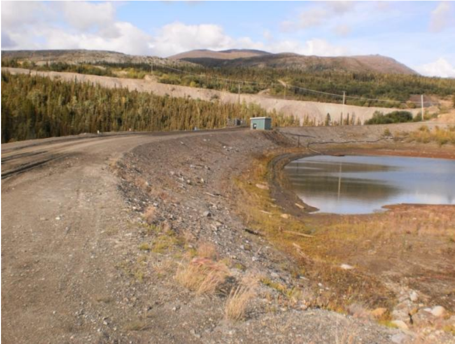
Photo 87 Dam crest/upstream slope and pond (August 23, 2011)
