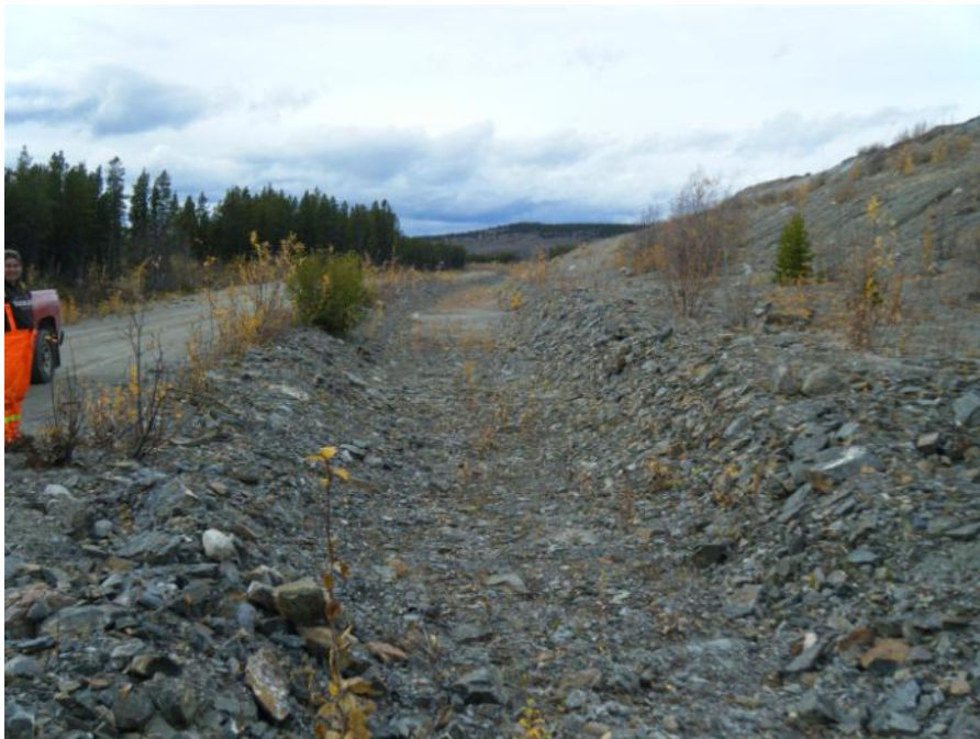
Photo 56 Vangorda Waste Dump Seepage Collection Ditch - looking downstream from Drain No. 1. (September 20, 2011)
