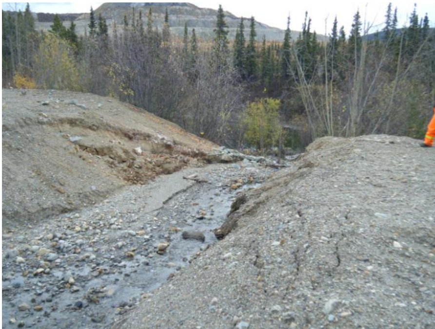
Photo 108 V-15 Diversion Ditch at its downstream end near Moose Pond (September 20, 2011)
