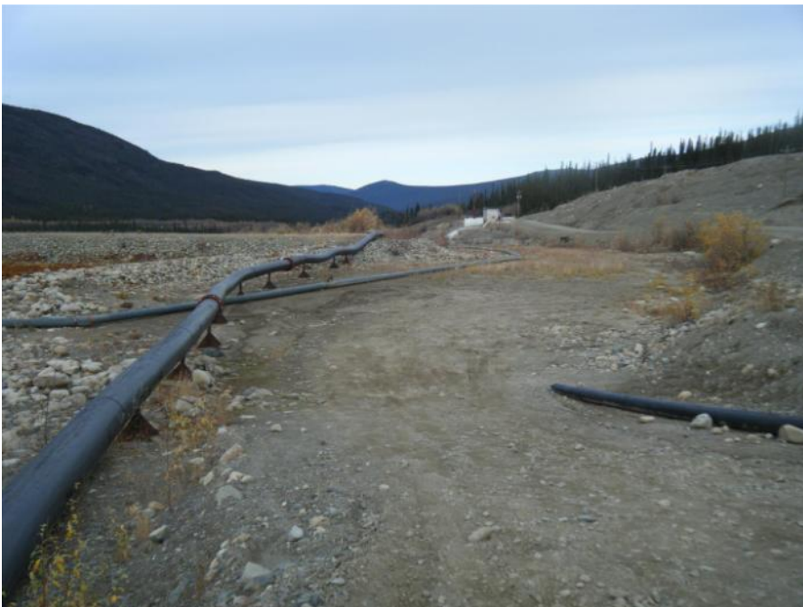
Photo 28 Intermediate Dam spillway channel - looking downstream (September 21, 2011)
