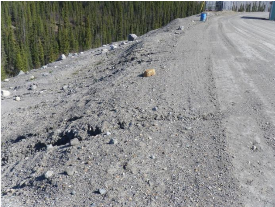
Photo 82 Dam crest and downstream slope (May 30, 2012)
