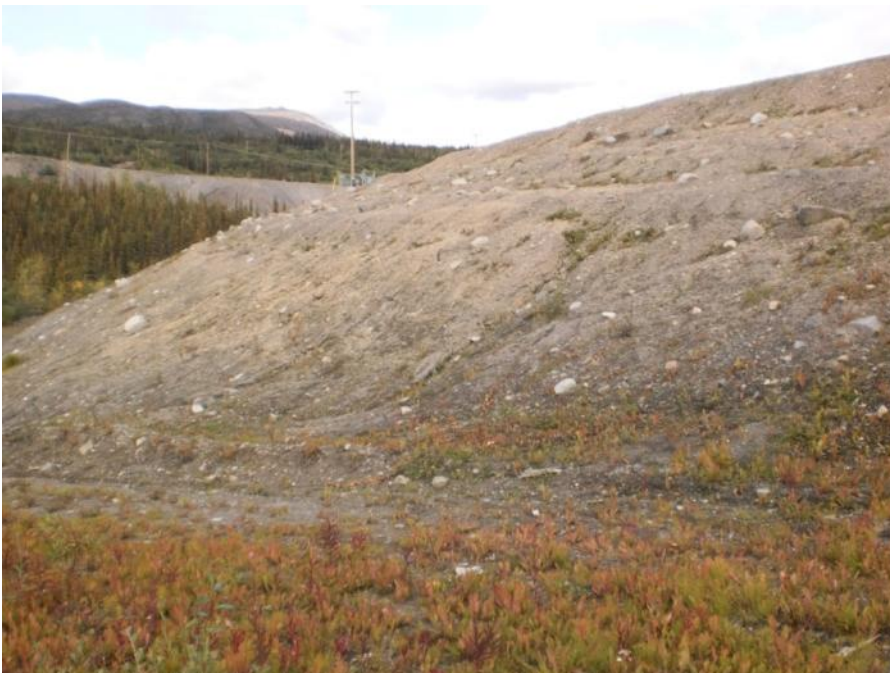
Photo 90 Downstream slope and berm (August 23, 2011)
