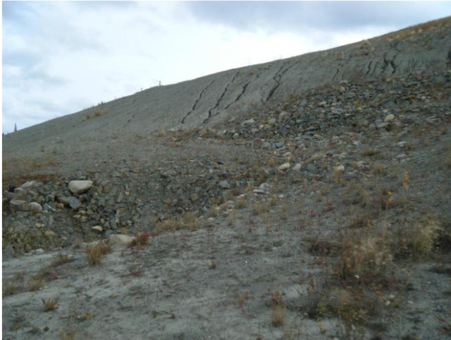
Photo 53 Vangorda Waste Dump at Drain No. 6 - showing previous subsidence of dump face (September 20, 2011)
