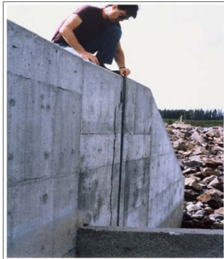
Figure 21 – Inspecting a spillway training wall
