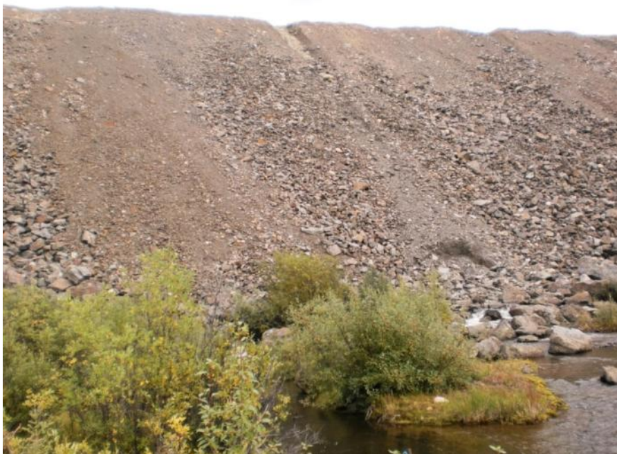
Photo 18 Downstream slope of Access Road between Faro and Vangorda Plateau (August 23, 2011)
