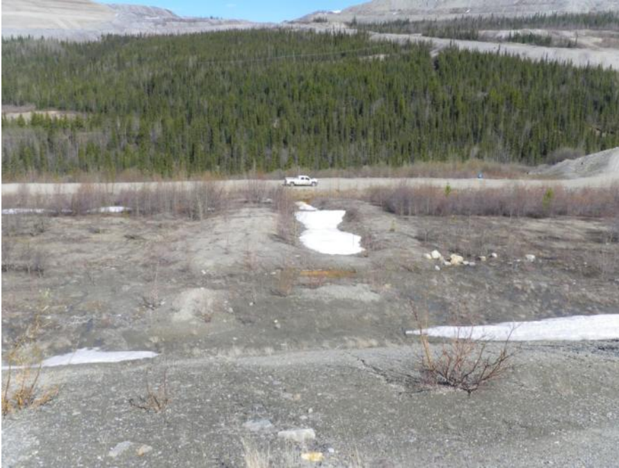
Photo 55 Dump slope and seepage collection ditch at drain no. 4 (May 30, 2012)
