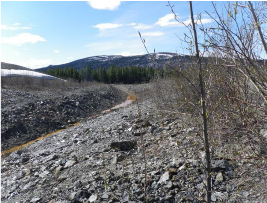
Photo 54 Seepage collection ditch between drain nos. 3 and 4. (May 30, 2012)
