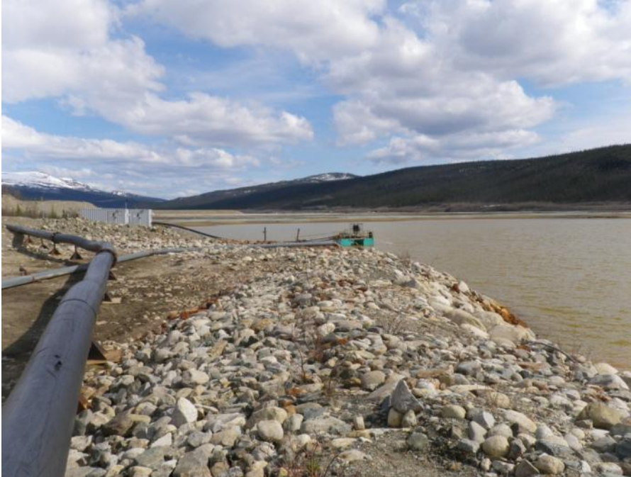
Photo 29 Intermediate Dam spillway at right abutment of dam looking upstream (May 29, 2012)
