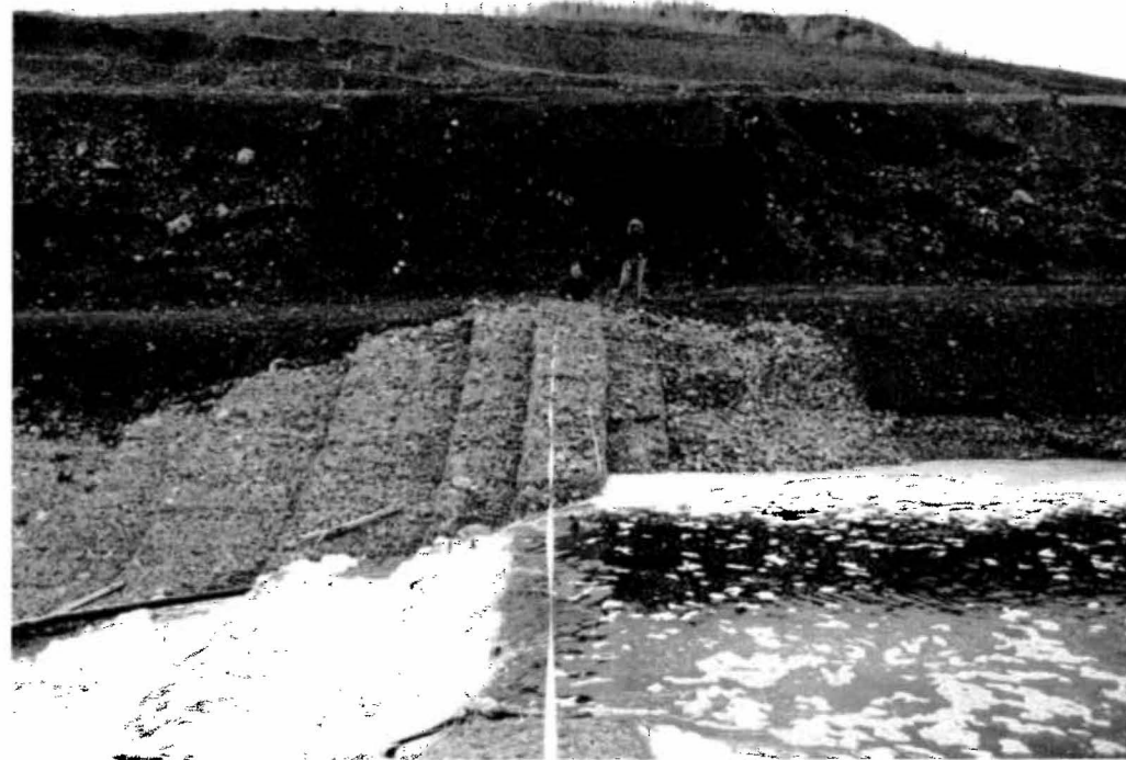
Photograph C1: Gabion drop structure - measurement location 1 across drawdown weir.
