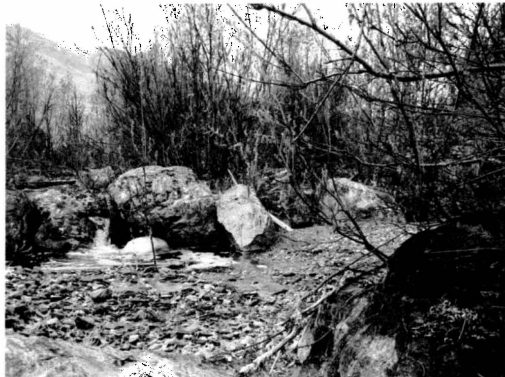
Photograph 6: Wolverine Creek - Rock lined channel: trees growing in channel and some sedimentation occurring.
