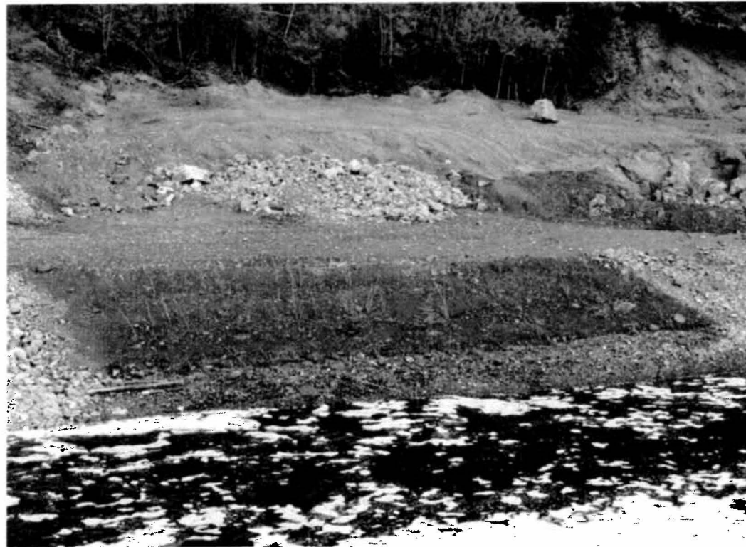
Photograph 3: High water line from spring freshet and vegetation planted on channel slopes.
