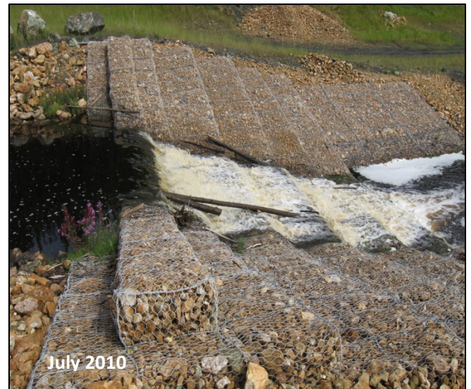
Figure 23 DS #2 Weir, Tier 5 and 6 in 2009 and cross channel view in 2010, view North
