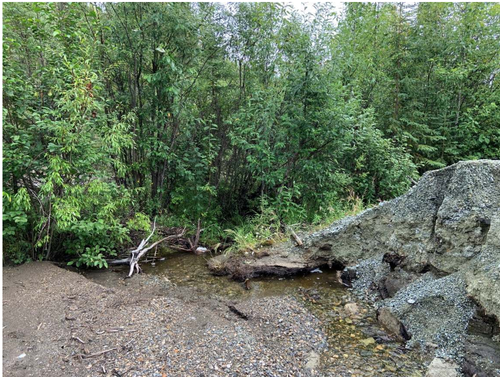
Appendix Photo 48. R11(H) – looking downstream.
