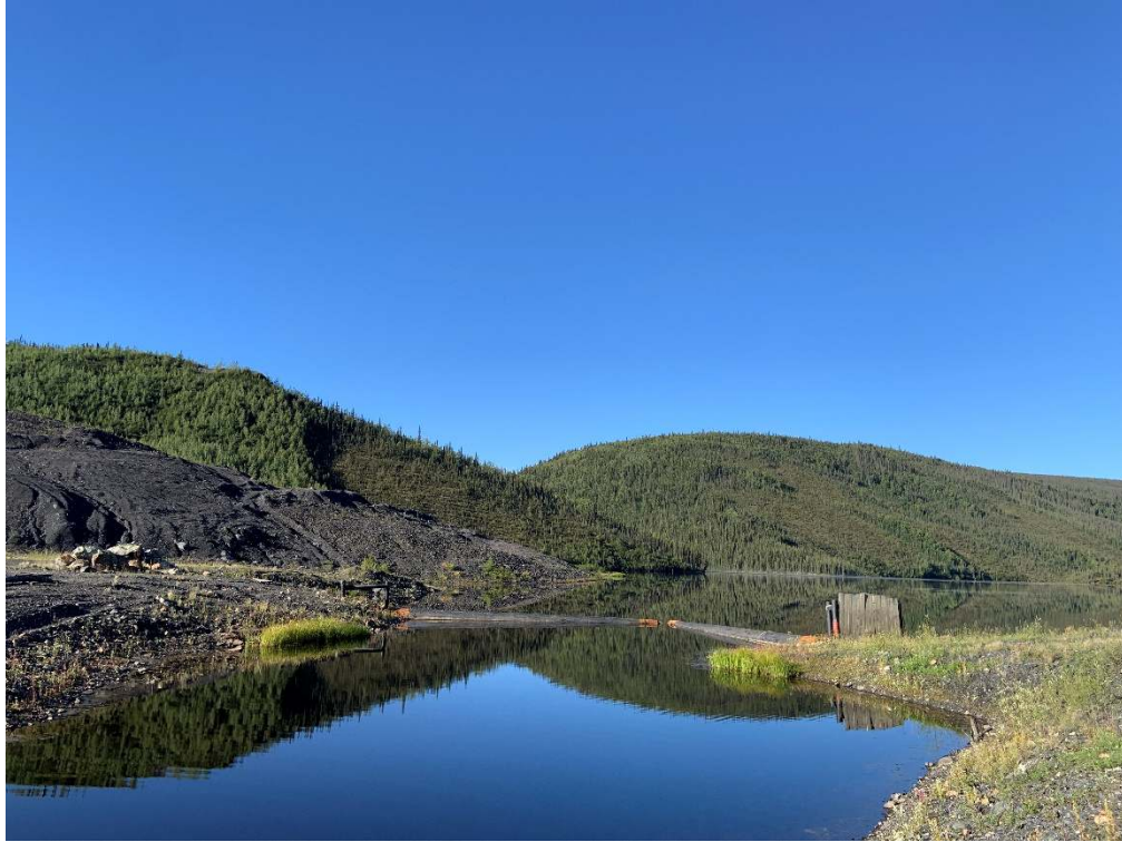
Appendix Photo 3. E1(H) – looking upstream.
