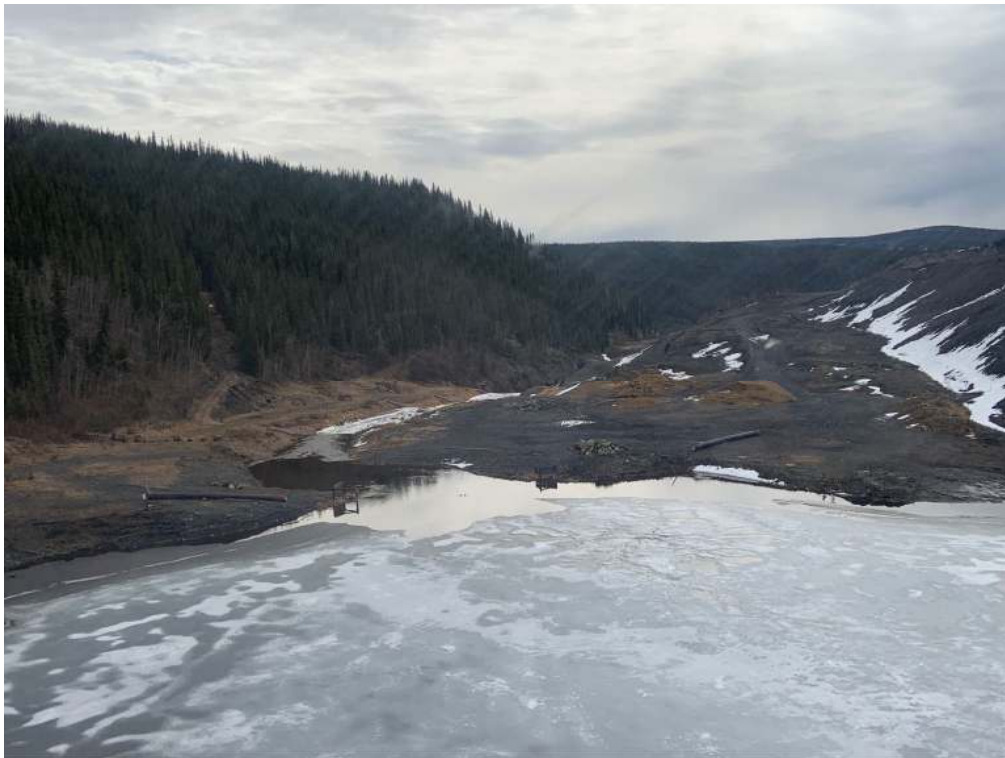
Appendix Photo 4. E1(H) – looking downstream.
