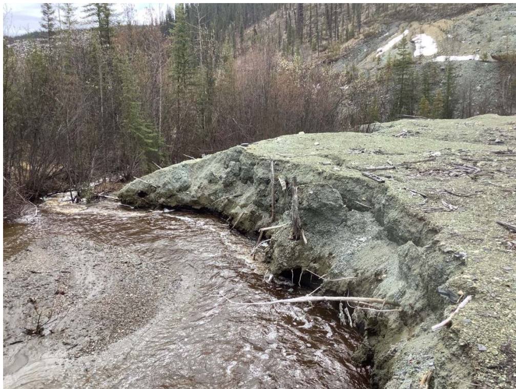
Appendix Photo 47. R11(H) – looking downstream.
