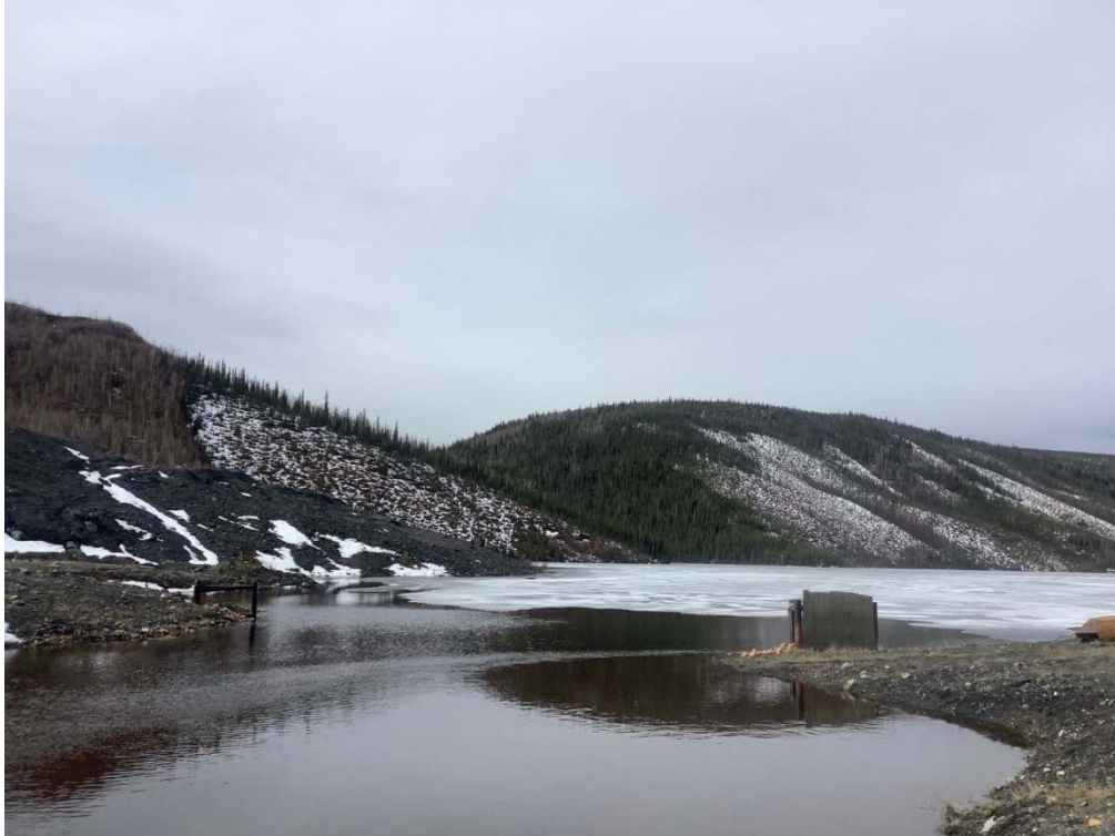
Appendix Photo 3. E1(H) – looking upstream.
