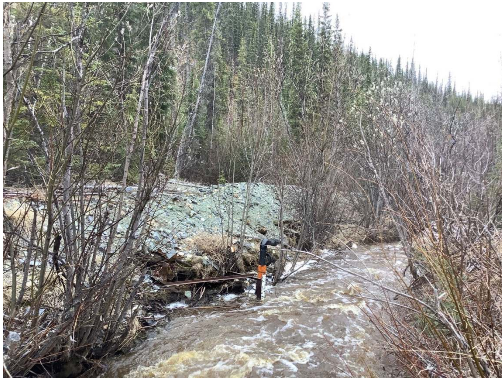
Appendix Photo 12. E3(H) – looking downstream.
