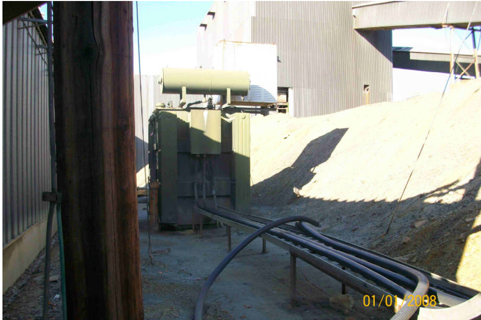
Grum Line Isolation Transformer and Cable Tray
