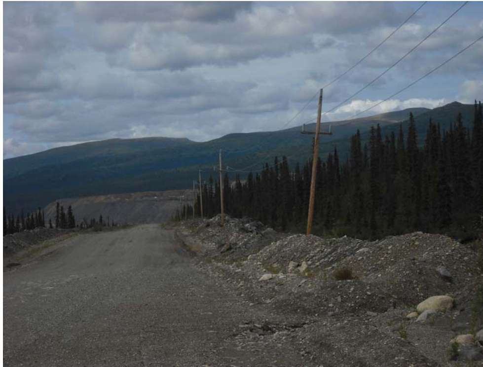
Typical Leaning Pole on 69 kV line – May be Straightened
