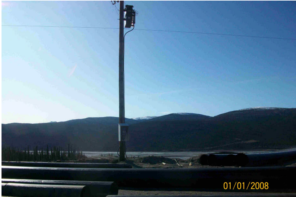
ETA Pole Configuration – Transformer will be moved by Arctic Power Drop and switch moved by Electrical Contractor
