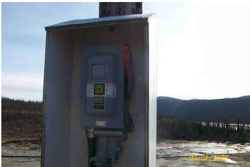
Existing ETA Fused Switch and Housing to be relocated to New Pole
