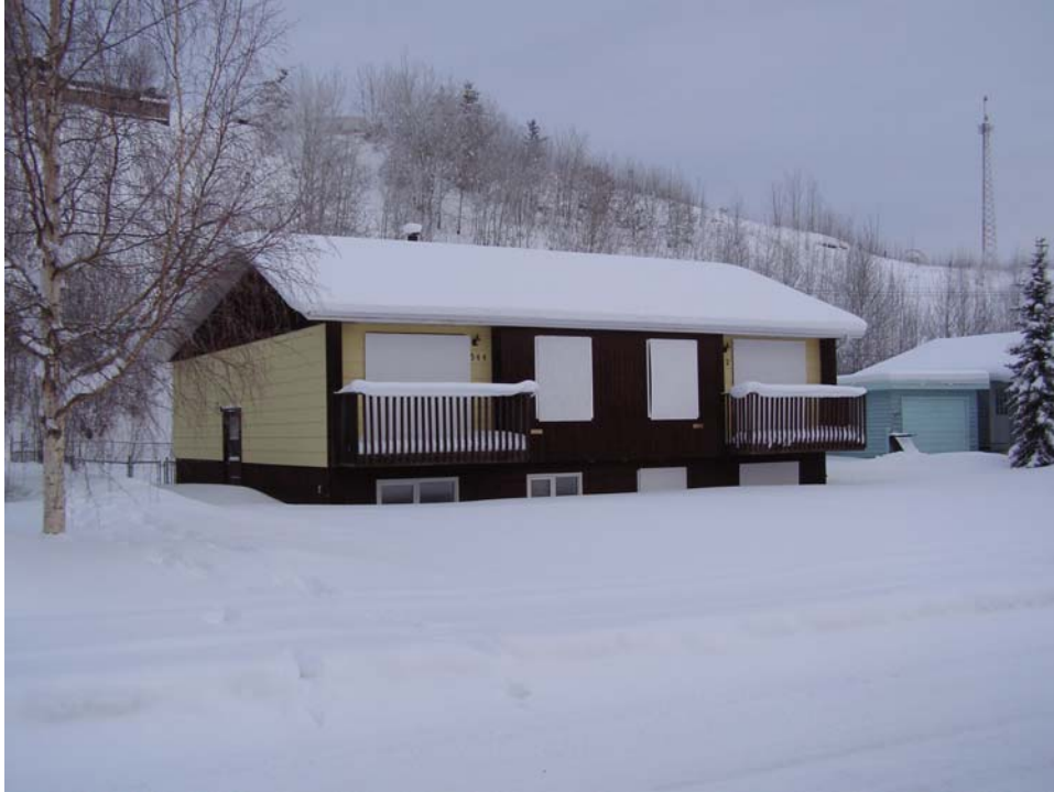
Photo 5 – Typical unoccupied duplex.
