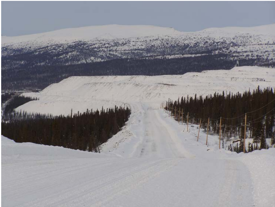
Photo 11 – Haul Road between Faro Mine and Vangorda/Grum site.
