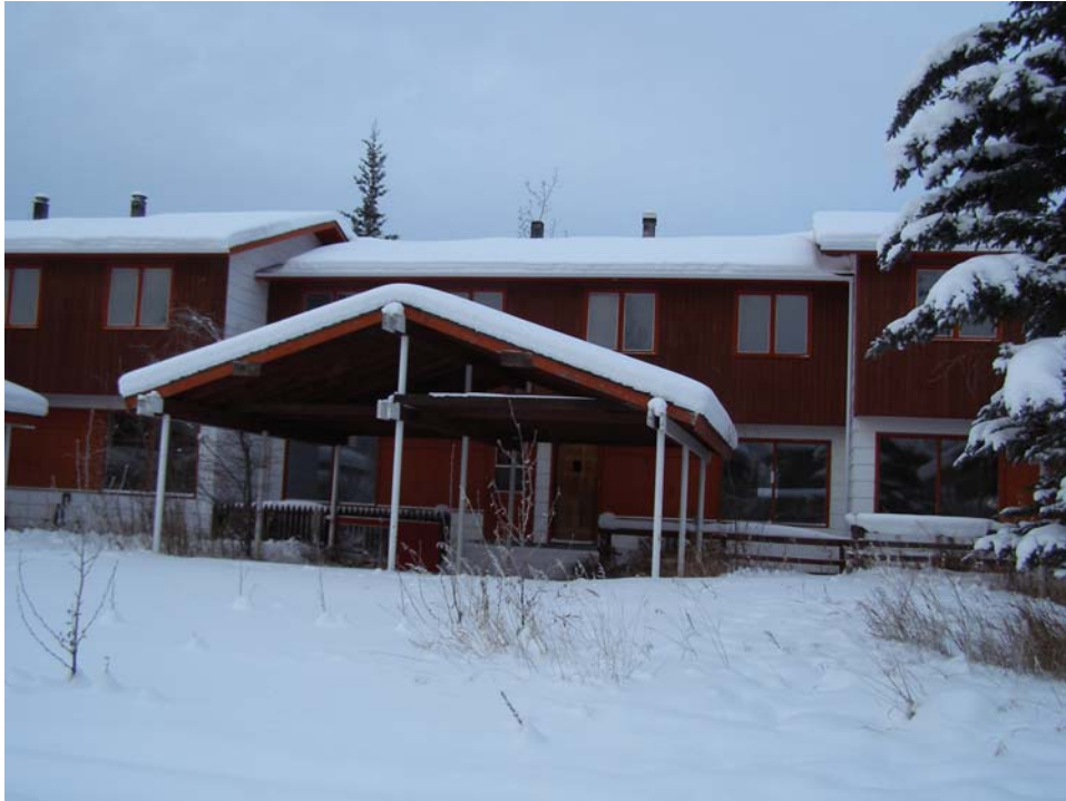
Photo 6 – Typical unoccupied row housing.
