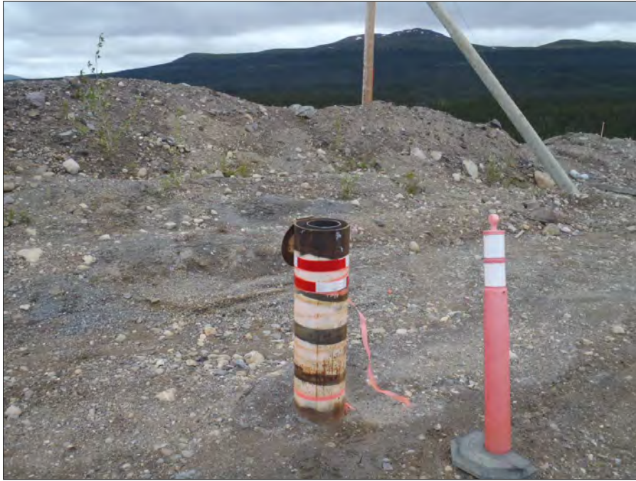
Photo 51: View of well PW14-01. Photo taken on June 17, 2015.
