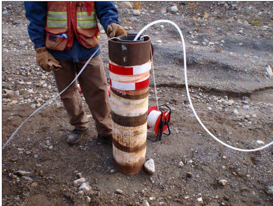
Photo 16: View of well PW14-01. Photo taken on September 11 th , 2015.
