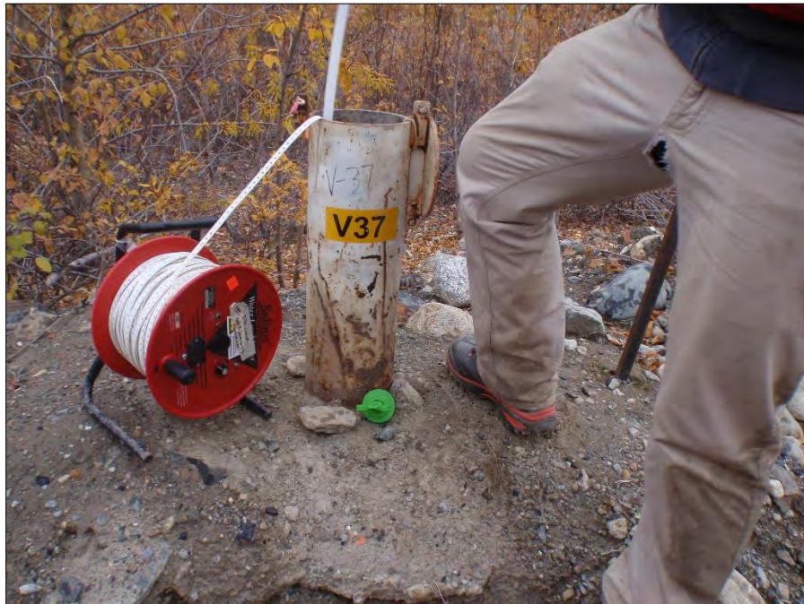
Photo 88: View of well V37. Photo taken on September 15 th , 2015.
