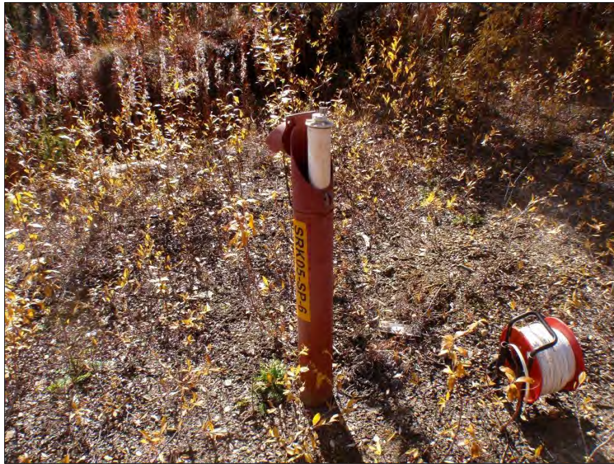
Photo 51: View of well SRK05-SP-6. Photo taken on September 11 th , 2015.
