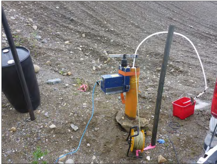
Photo 15: View of well X24-96D. Photo taken on June 2 nd , 2016.
