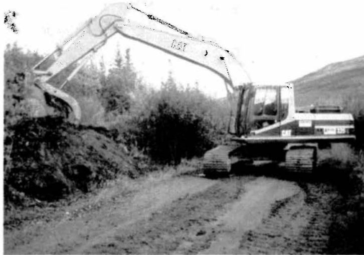
Photo 5: Excavator filling open Bellekeno hole.
