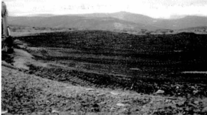
Photo 3: View of Shamrock J vent shaft filled and mounded with building removed.
