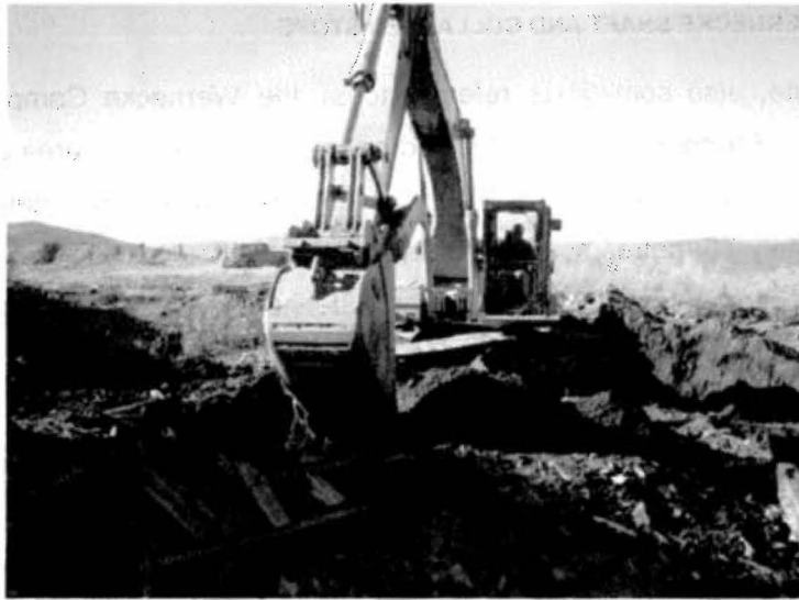
Photo 7: View of Wernecke shaft being filled.
