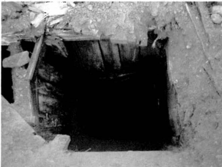
Photo 6: View of Wernecke shaft building located below the manager's house at the base of the hill.
