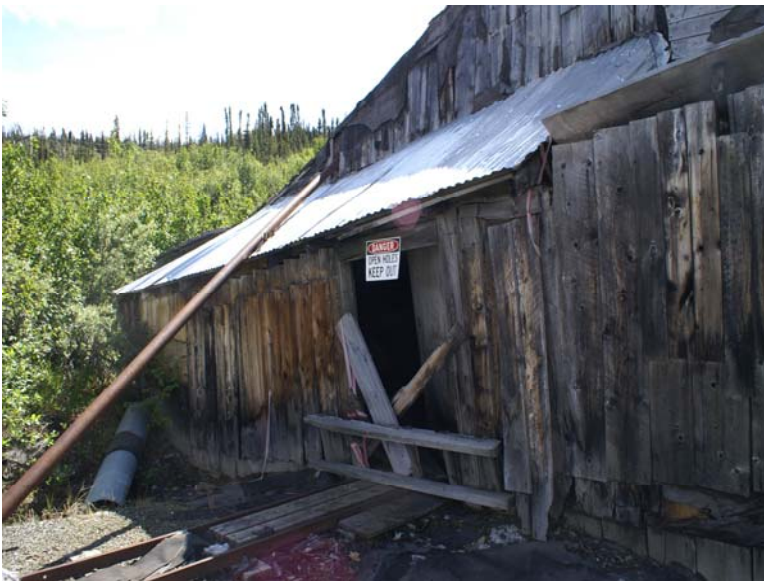
Plate 3: Brefalt Shafthouse - Before
