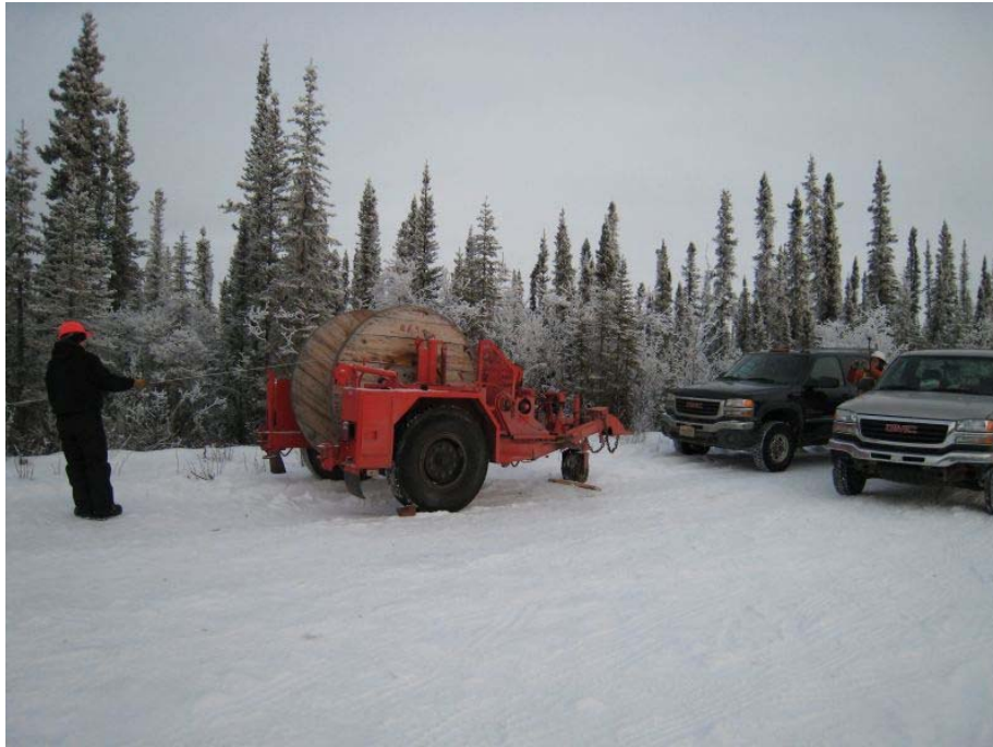
Labourer helping to feed line onto wire spooler in the Tailings to McQuesten River Area.
