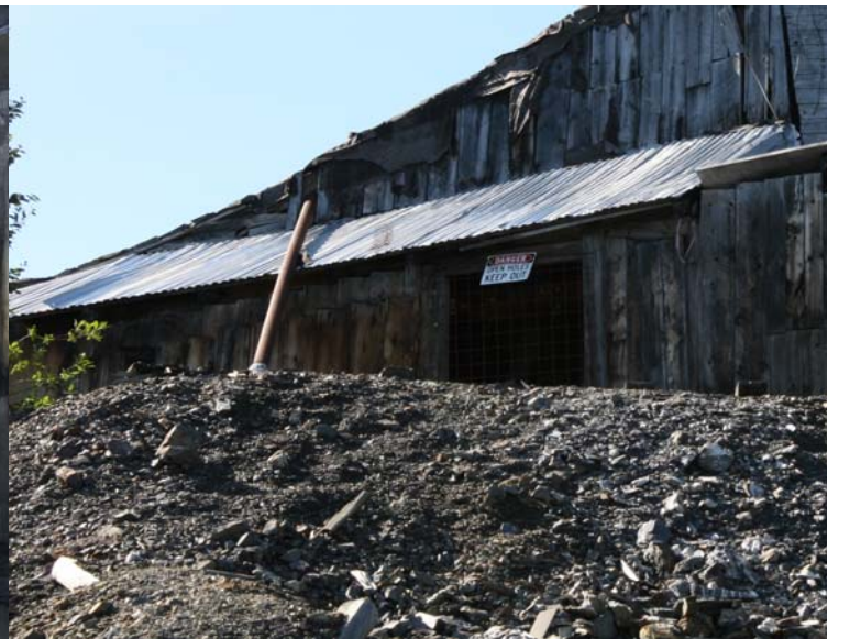
Plate 4: Brefalt Shafthouse - After
