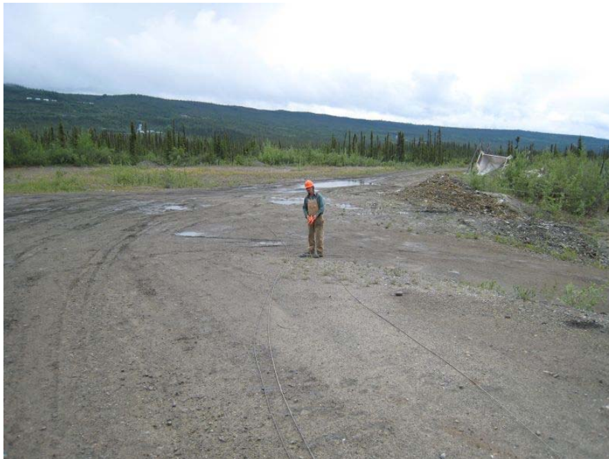
Picture of personnel hand rolling wire in the Tailings Dam Area
