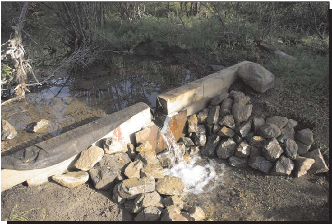
Photo 6 Weir 4 at North Dam. Photo taken Aug. 6, 2008
