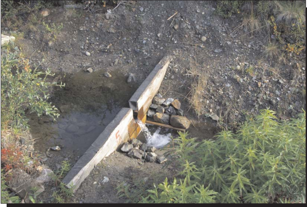
Photo 3 Weir 5 at South Dam. Photo taken Aug. 6, 2008
