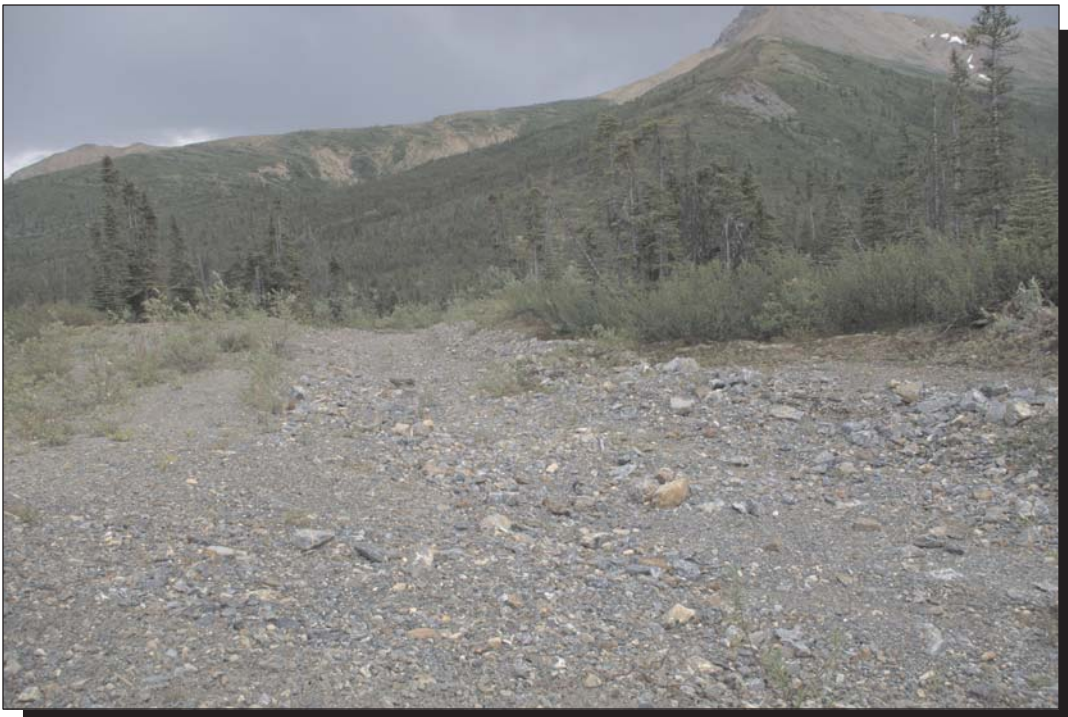
Photo 2 Emergency Spillway on South Dam. Aspect: E. Photo taken Aug. 6, 2008
