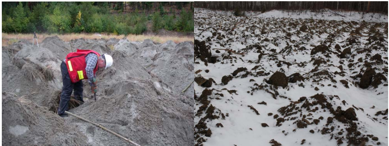
Photo 3. Examples of ‘Rough and Loose’ surface preparation at other sites. Left: tailings area in southern British Columbia (photo – Altura); Right: platform in central Alberta illustrating the ‘snow-trap’ effect in depressions (photo – Polster Environmental Services Ltd.)
