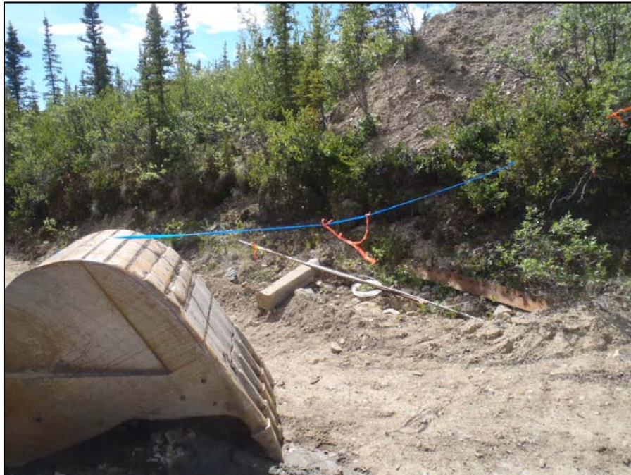
Photo 34: View of well GSI-PC-01A and GSI-PC-01B. Wells have been destroyed by excavator due to area being part of an active Placer Mine. Photo taken on June 27, 2014.
