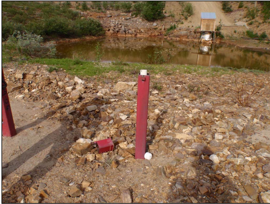
Photo 57: View of well MW09-20. Photo taken on June 28 th , 2014.
