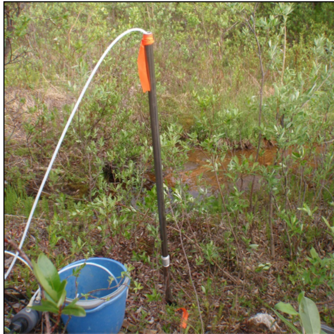
Photo 10: View of drive point well GSI-HA-01A. Photo taken on June 27 th , 2014.
