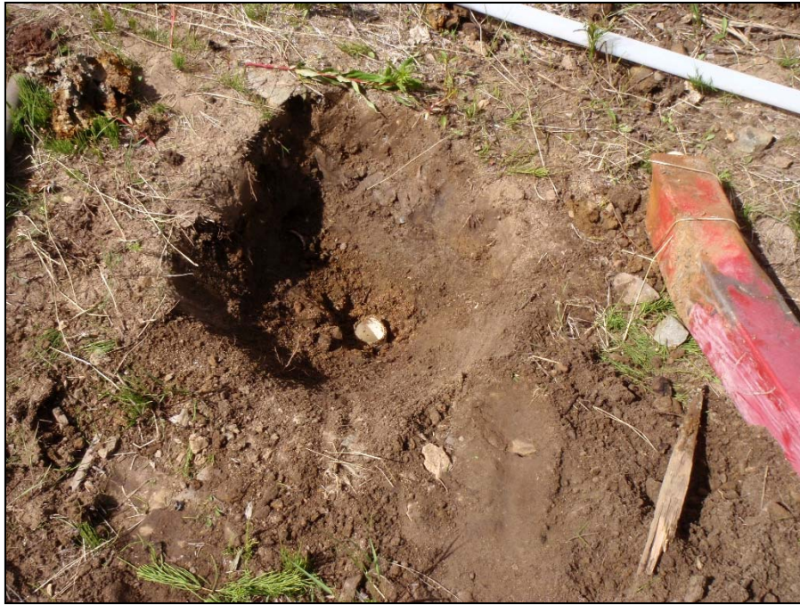
Photo 17: View of the first step of well repair for well MW09-17. A hole was excavated around well to the top of where the stick-up was broken. Photo taken on June 28 th , 2014.
