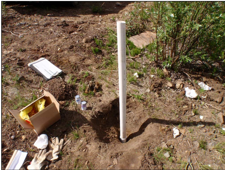
Photo 18: View of the second step during well repair for well MW09-17. A cup-link and new PVC pipe were attached. Photo taken on June 28 th , 2014.
