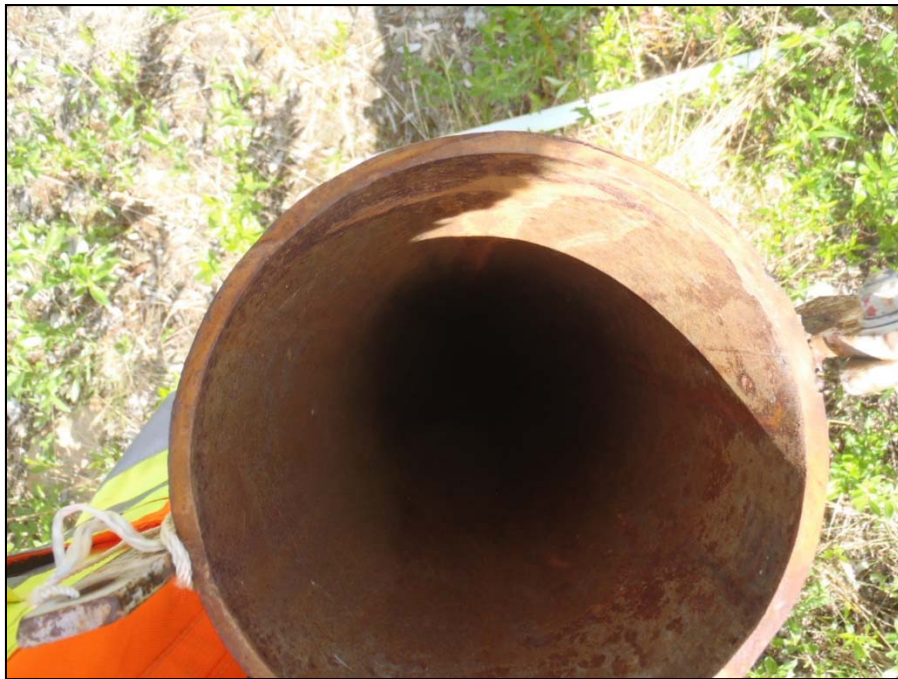
Photo 30: View of well GLL07-02 showing the absence of a stick-up. Photo taken on June 28 th , 2014.
