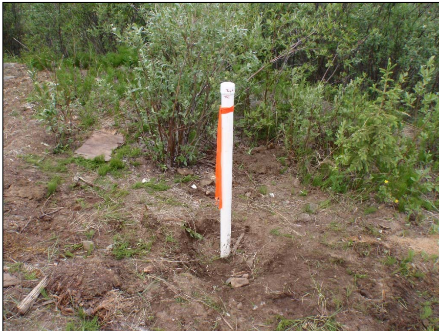
Photo 20: View of the fourth step during well repair of well MW09-17. The bentonite seal was covered with soil and well redeveloped manually using watterra tubing. Photo taken on June 28 th , 2014.
