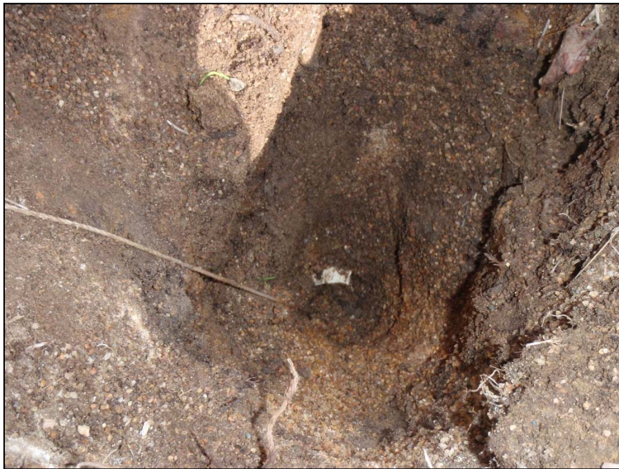
Photo 16: View of damaged well MW09-17. Existing bailer stuck in well due to large amount of soil that had fallen into well. Photo taken on June 26 th , 2014.
