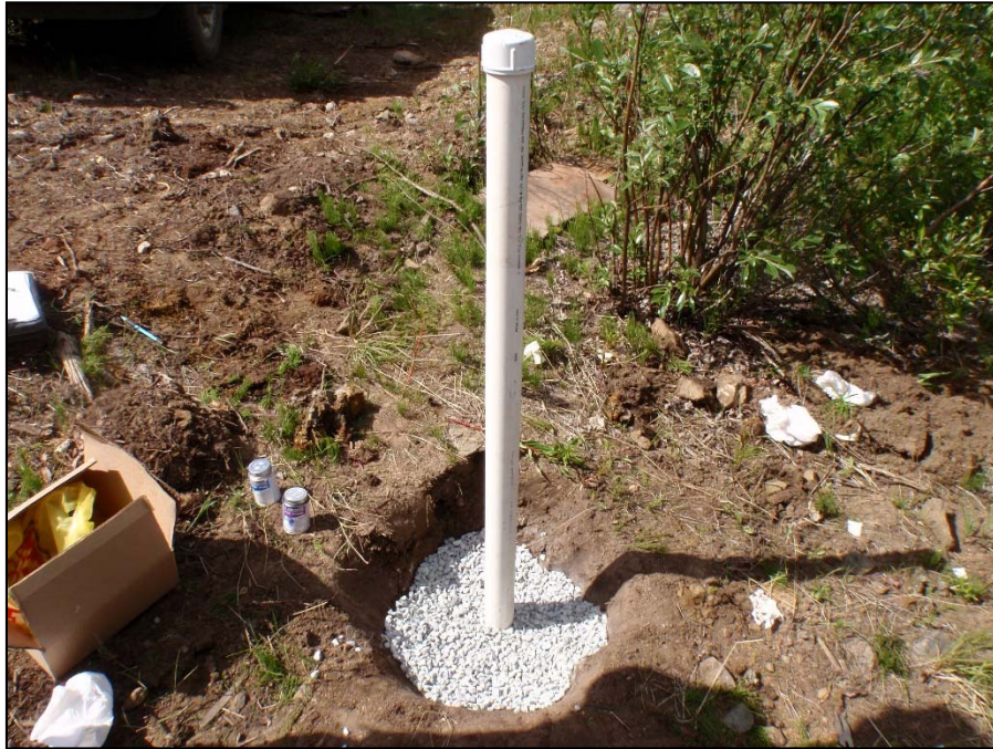
Photo 19: View of the third step during well repair for well MW09-17. Bentonite chips were used to seal the previously dug hole around stick-up. Photo taken on June 28 th , 2014.
