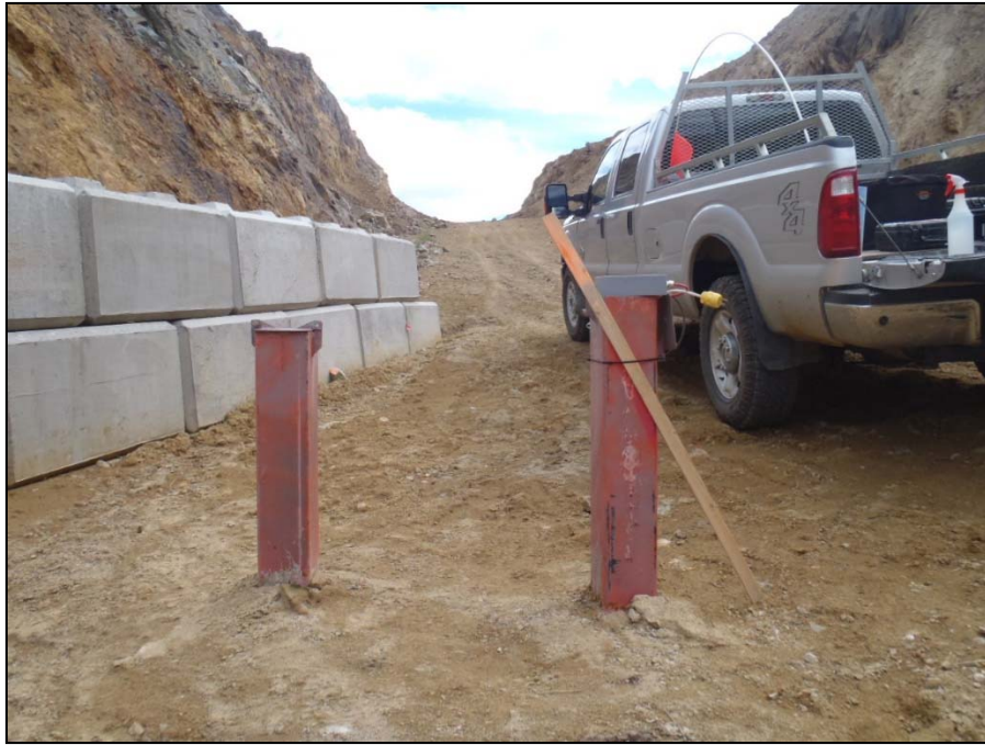
Photo 27: View of well CH-P-13-05/50. Photo taken on June 26 th , 2014.
