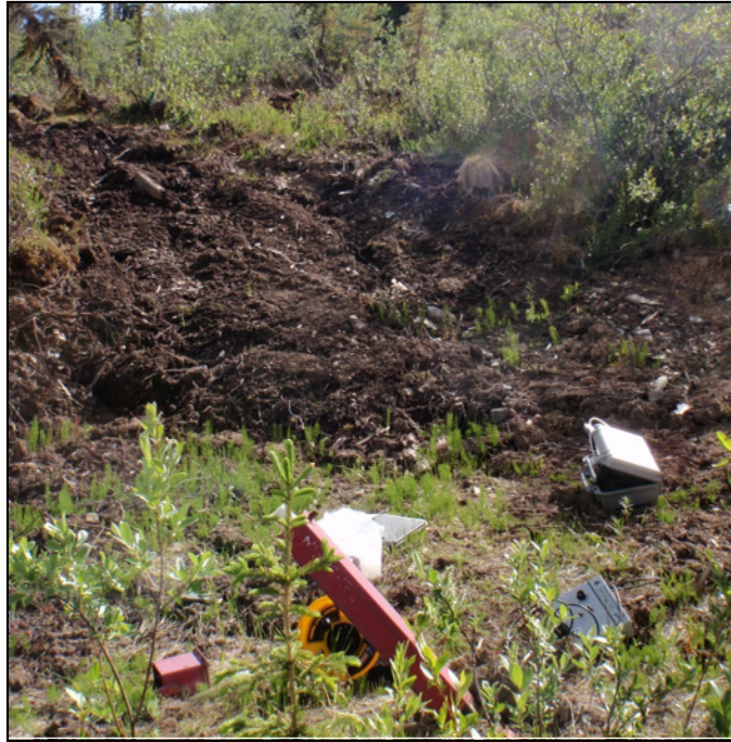
Photo 15: View of well MW09-17. Stick-up and steel monument broken upon arrival at site. Loose earth up earth above well suggests excavator could have damaged the well. Photo taken on June 26 th , 2014.
