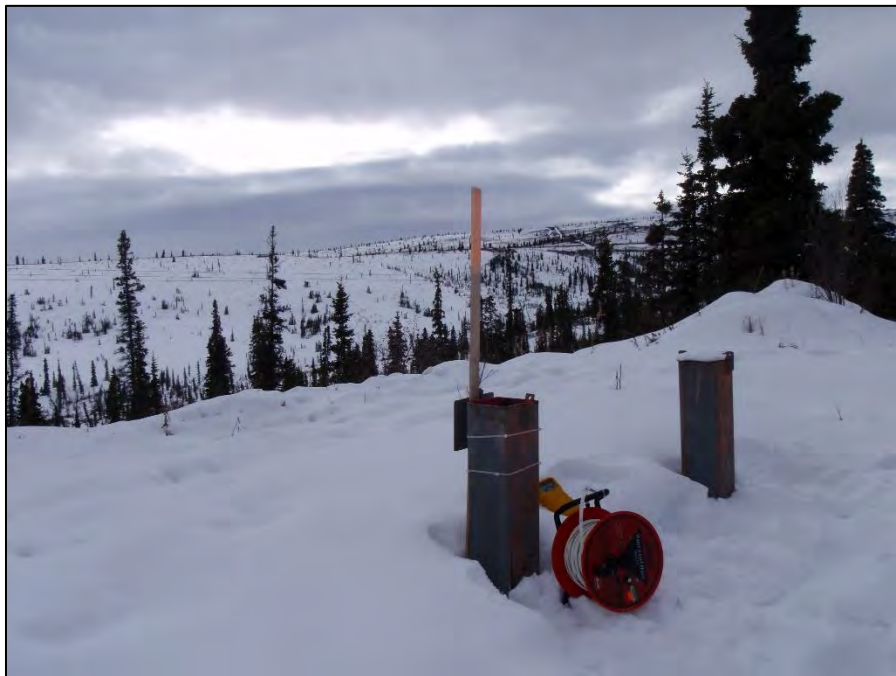
Photo 56: View of well CH-P-13-02/10. Photo taken on March 19, 2015.
