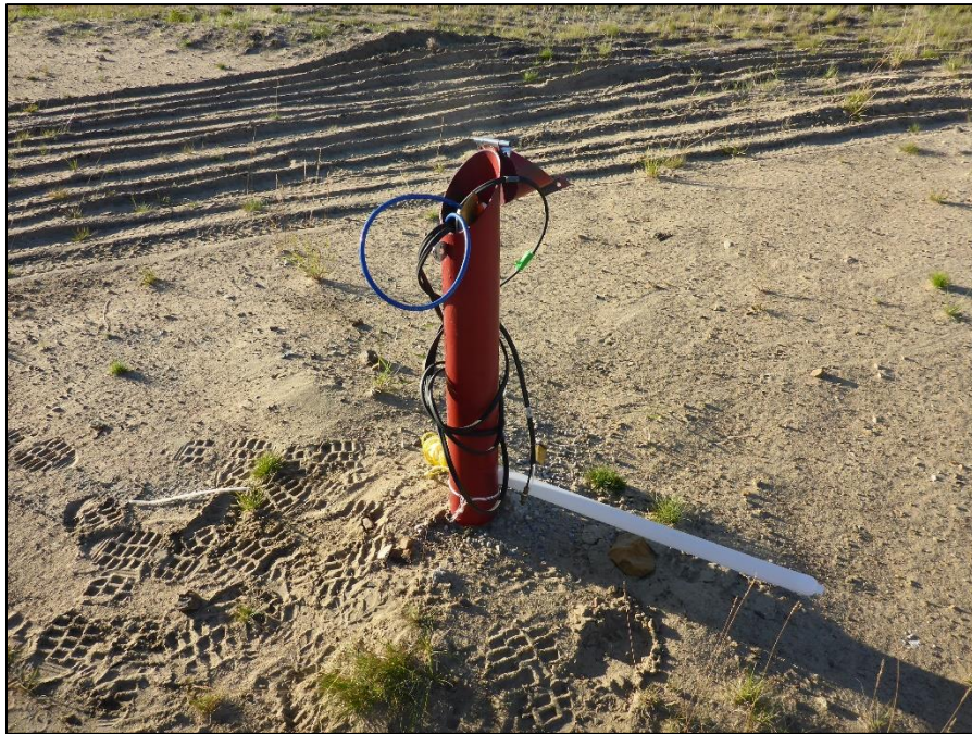
Photo 33: View of well W14103083BH04. Photo taken on August 30, 2016.
