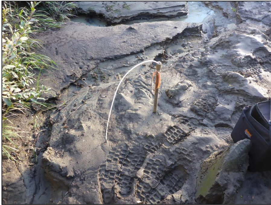
Photo 29: View of drive point well MP09-03. Photo taken on August 31, 2016.
