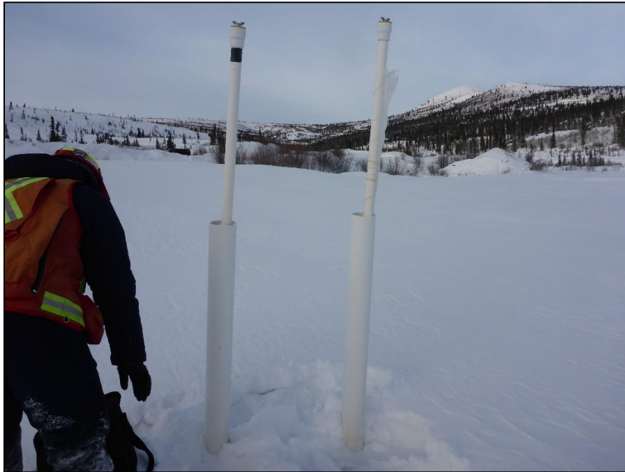
Photo 37: View of wells MP09-11 and MP09-12. Photo taken on January 31, 2017.
