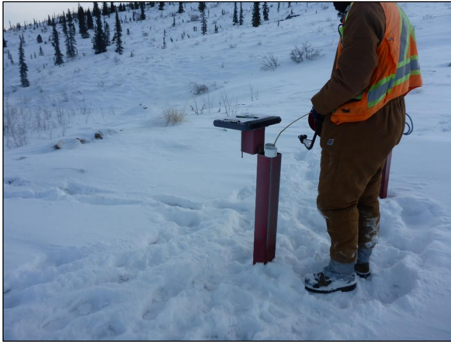
Photo 45: View of well MW09-20. Photo taken on January 31, 2017.
