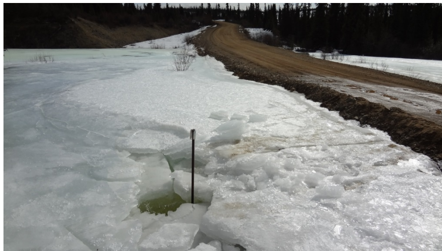
Photo 19. Overview of Vicotira Creek at Road (WQ-VC-R in background) showing overflow ice conditions, and secondary culvert in foreground.
