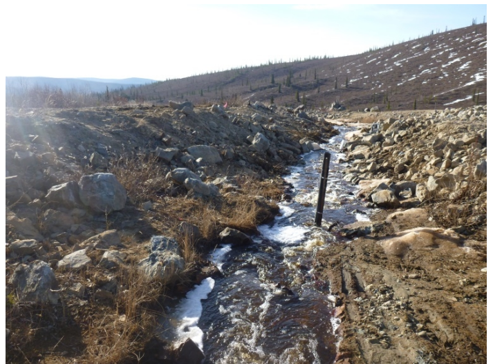
Photo 12. H-DC-B, looking downstream (May 14, 2015).
