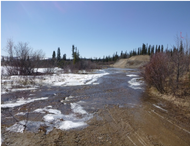
Photo 37. H-VC-R, looking at water ponding in parking area (stilling well in channel) (May 4, 2015).
