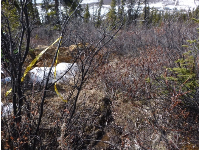
Photo 76. WQ-WR-SEEP-A looking downstream at seepage area (May 6, 2015).
