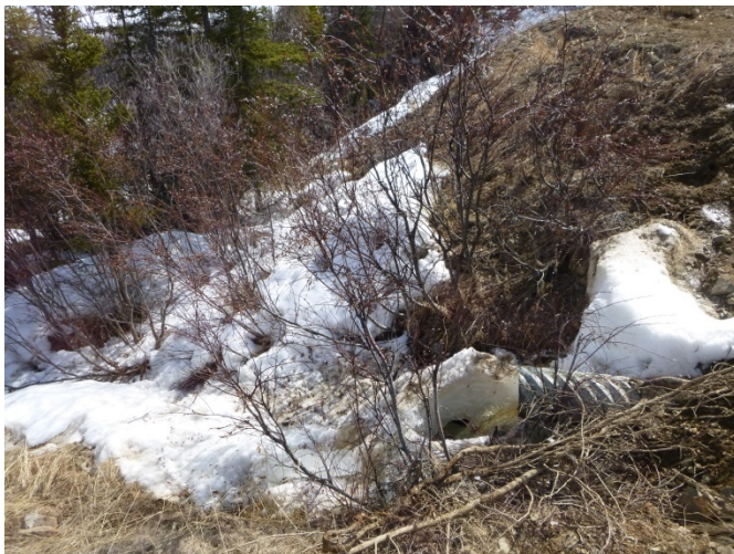
Photo 42. H-PC-DSP, looking across at culvert outlet (May 5, 2015).
