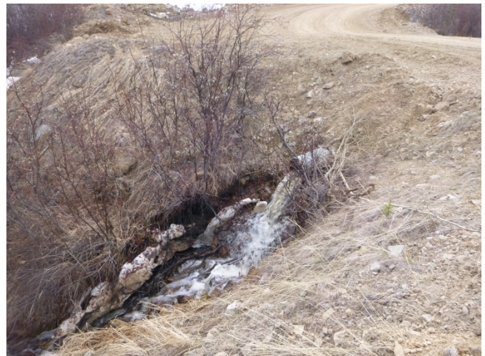
Photo 43. H-PC-DSP, looking across at culvert outlet (May 12, 2015).
