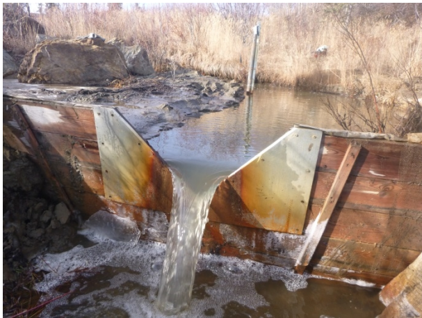
Photo 7. H-DC-M WP – looking upstream showing accumulated sediment.
