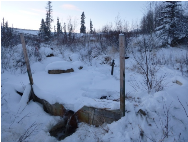
Photo 7. H-DC-M WP – looking upstream. Ice removed from outlet of weir.
