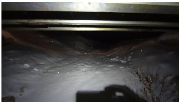
Photo 3. H/WQ-DC-B – looking downstream. Site frozen to bed.
