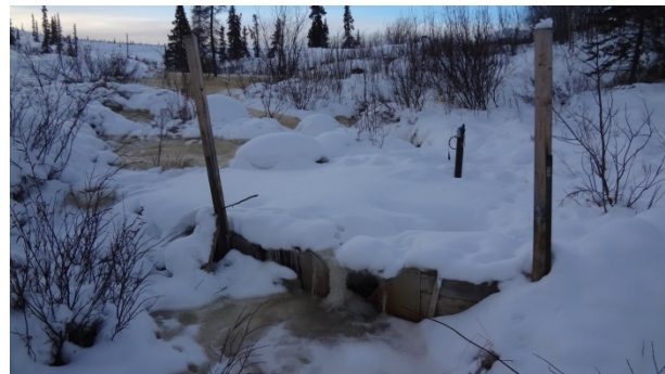
Photo 4. H-DC-M WP – looking at weir pond, showing seepage upstream of pond extending from seepage discharge.
