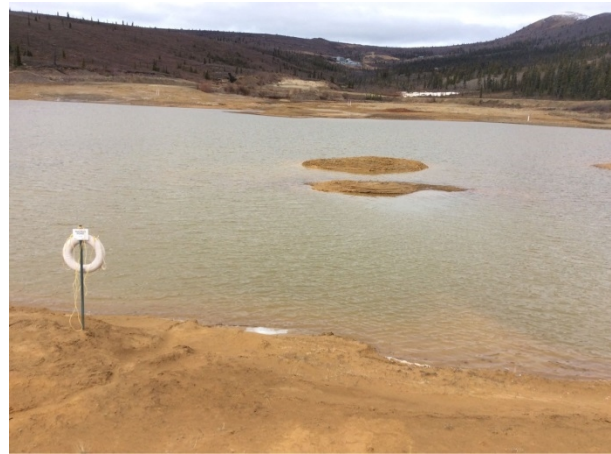
Photo 12. WQ-TP –overview of tailings pond.
