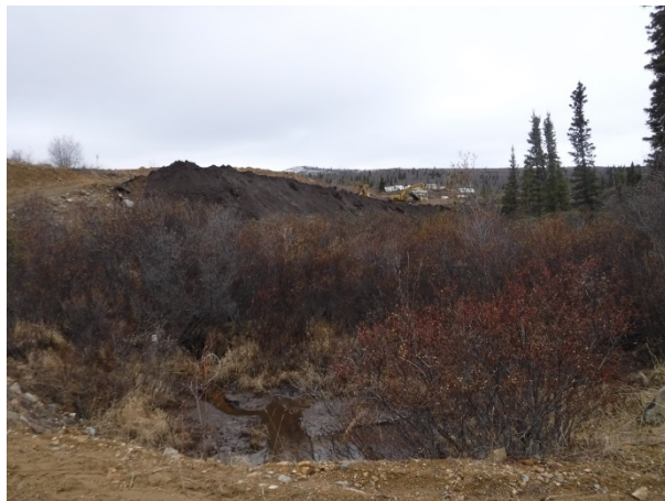
Photo 21. Placer mining works upstream of WQ-PC-U.
