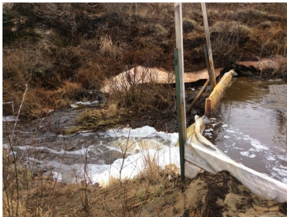
Photo 15. H-DC-M WP – overview of weir pond.
