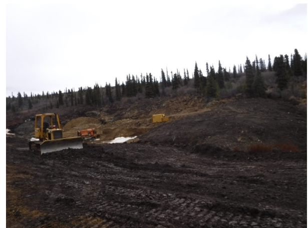
Photo 22. Placer mining works upstream of WQ-PC-U.
