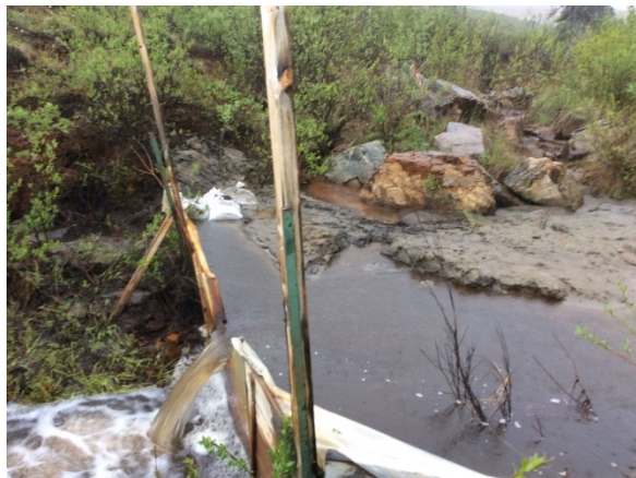
Photo 15. H-DC-M WP – overview of weir pond.
