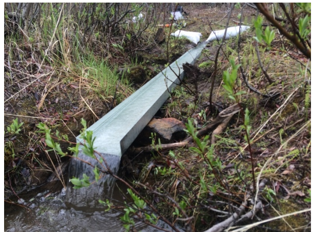
Photo 2. H/WQ-DC-DX+105 – looking upstream at trough installed for volumetric measurements.
