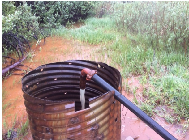
Photo 14. H/WQ-SEEP – looking downstream.
