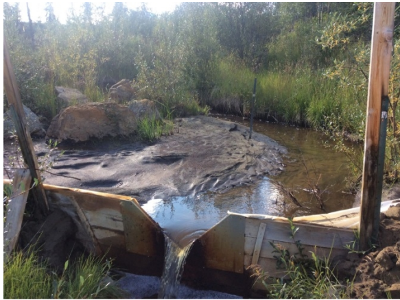
Photo 13. H-DC-M WP – looking upstream at weir pond.
