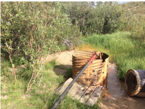
Photo 11. H/WQ-SEEP – looking downstream.
