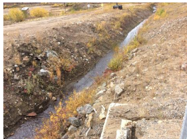
Photo 6. WQ-DC-B – overview, looking upstream
