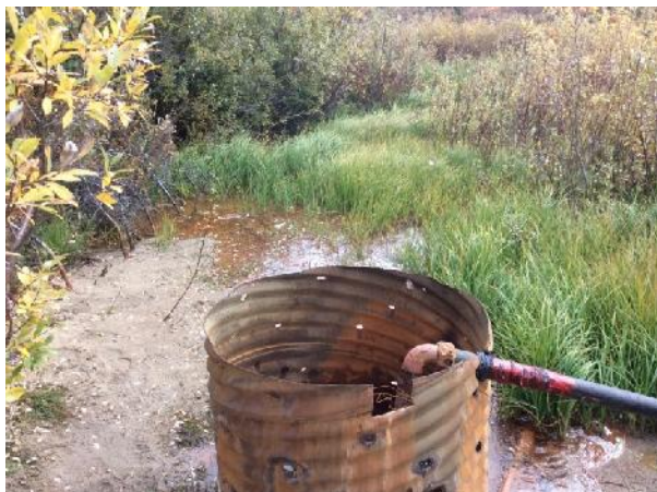
Photo 11. H/WQ-SEEP – looking downstream.
