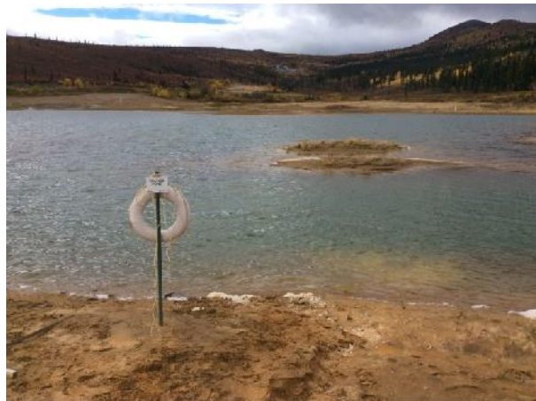
Photo 9. WQ-TP – overview of tailings pond.
