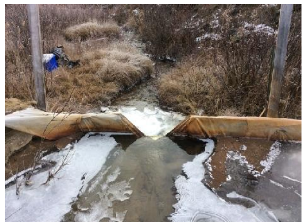
Photo 12. H-DC-M WP – looking downstream from weir pond.
