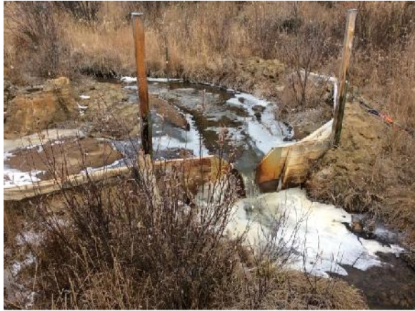
Photo 13. H-DC-M WP – overview of weir.
