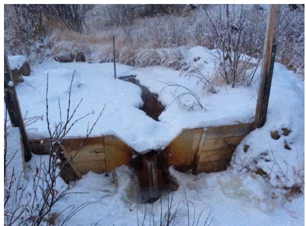
Photo 12. H-DC-M WP – looking upstream at weir pond.
