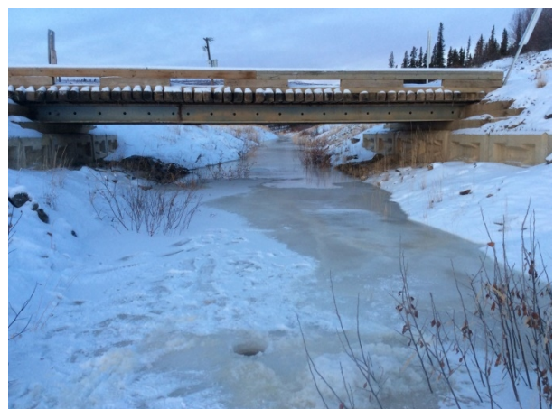
Photo 6. WQ-DC-B – looking upstream.
