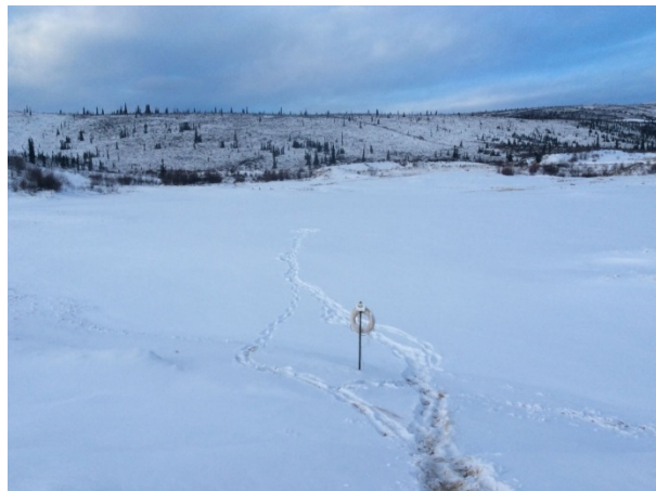
Photo 9. WQ-TP – overview of tailings pond.
