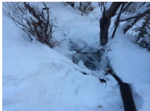
Photo 24. WQ-PW – looking downstream of pipe.
