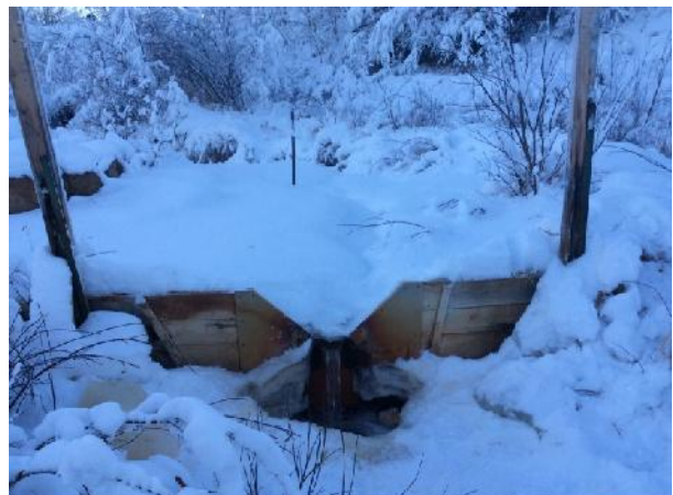
Photo 8. H-DC-M WP – looking upstream at weir pond.
