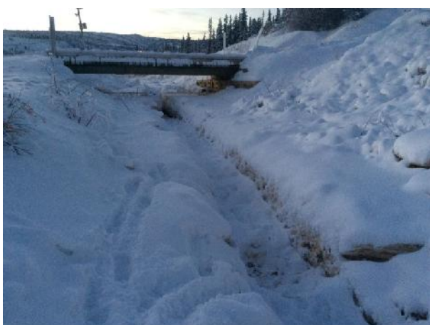
Photo 3. H/WQ-DC-B – looking upstream (site dry).
