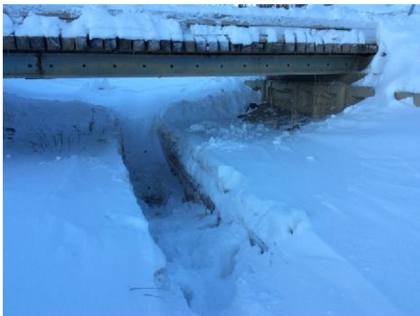
Photo 3. H/WQ-DC-B – looking upstream (site dry).
