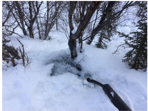
Photo 22. WQ-PW – pipe outlet.
