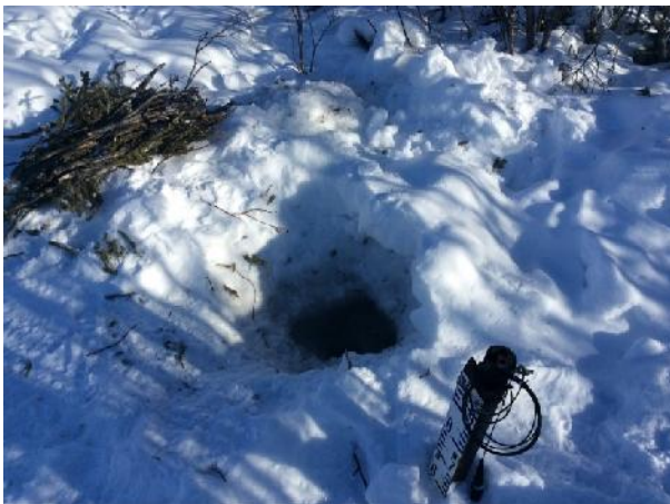
Photo 21. H-VC-R+290 – overview of stilling well.
