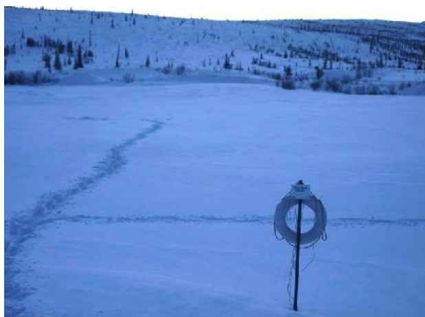
Photo 5. WQ-TP – overview of tailings pond.
