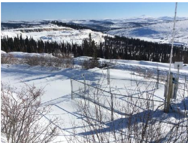
Photo 23. Meteorological Station overview
