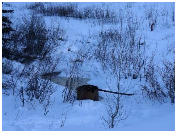
Photo 7. H/WQ-SEEP – looking downstream at discharge site.
