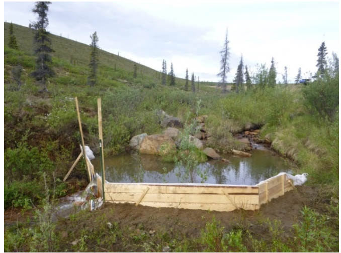
Photo 6. New weir construction at H-DC-M, looking upstream (June 24, 2014).
