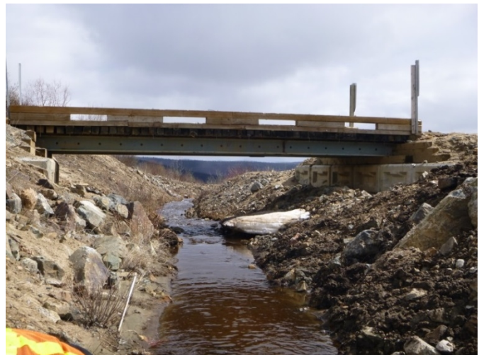
Photo 4. WQ-H-DC-B, looking downstream from WQ-DC-B site towards H-DC-B station (May 21, 2014).
