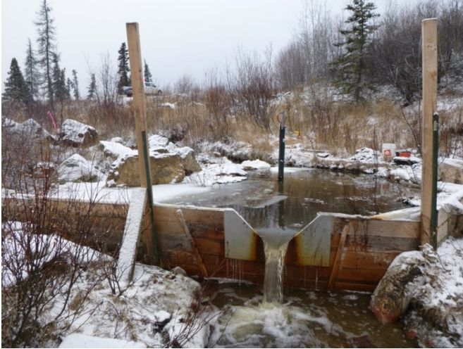
Photo 9. H-DC-U WP looking upstream (October 15, 2014).
