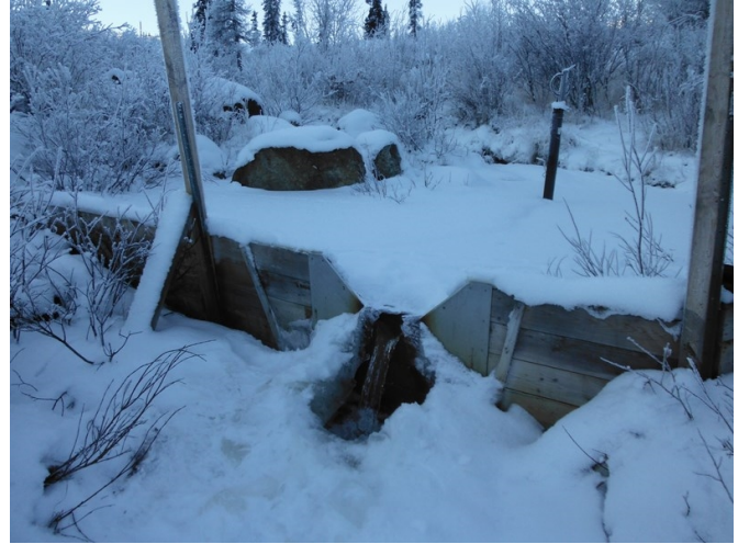
Photo 10. H-DC-M WP looking upstream at weir pond (November 12, 2014).
