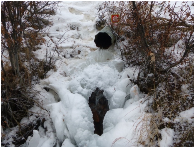
Photo 26. H-PC-DSP culvert looking upstream (October 14, 2014).
