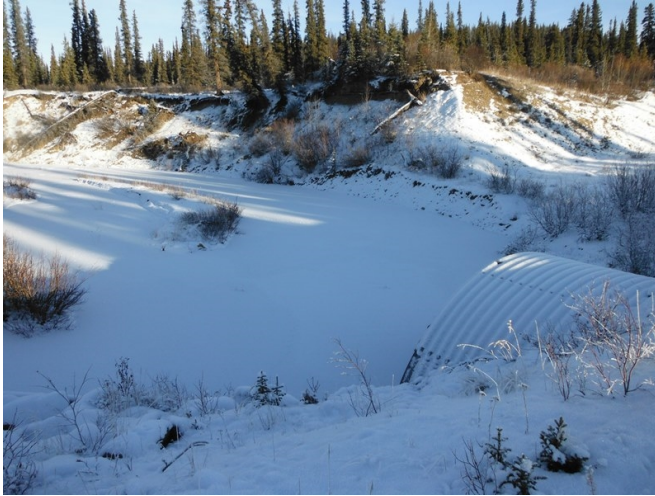
Photo 21. WQ-VC-R looking upstream from road crossing (November 12, 2014).
