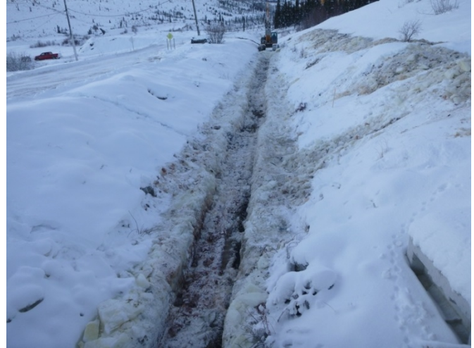
Photo 6. Diversion channel being dredged upstream of WQ-DC-B (December 15, 2014).
