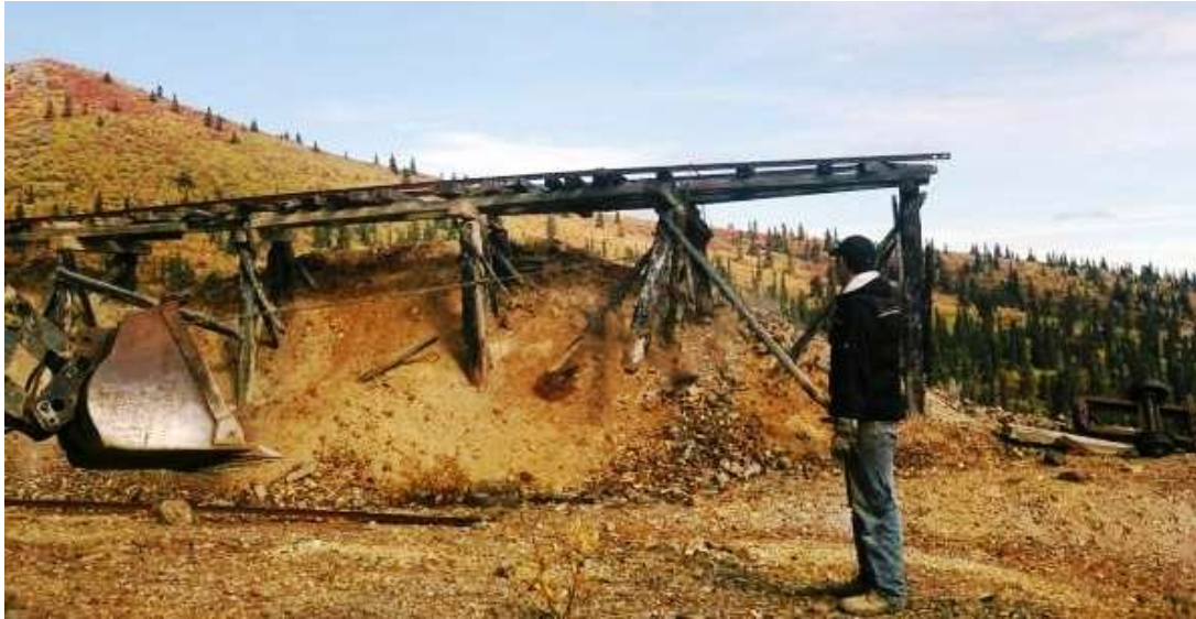
Removal of Debris and Salvage Materials
