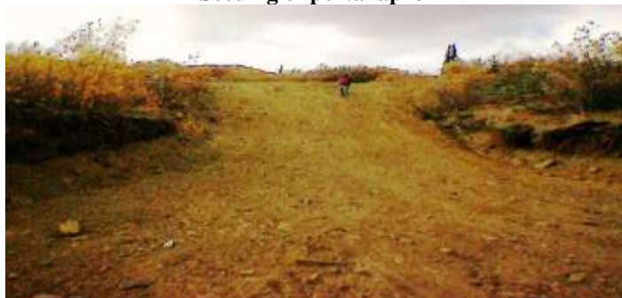
Seeding of portal apron
