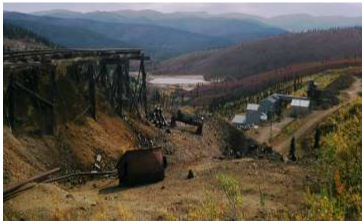
Portal Area – Rail Removal
