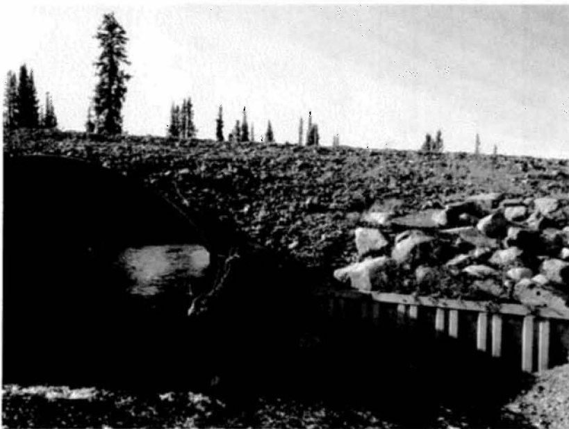
Figure 2. Gabion baskets were also installed on the right hand side of the culvert under the road bed material. Note the large tree stuck in the culvert in the foreground.
