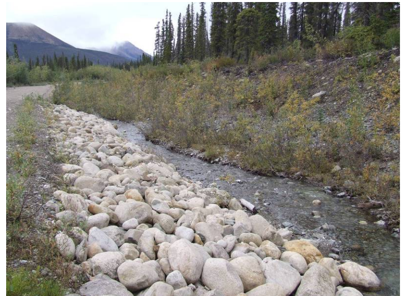
Photo #16; NWID looking downstream.
