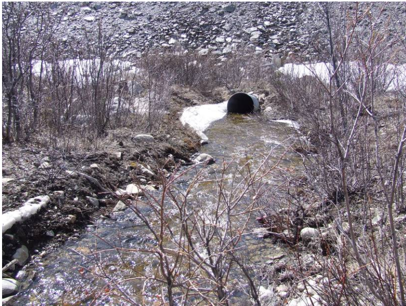
VR, looking downstream to haul road, May 30, 2012.
