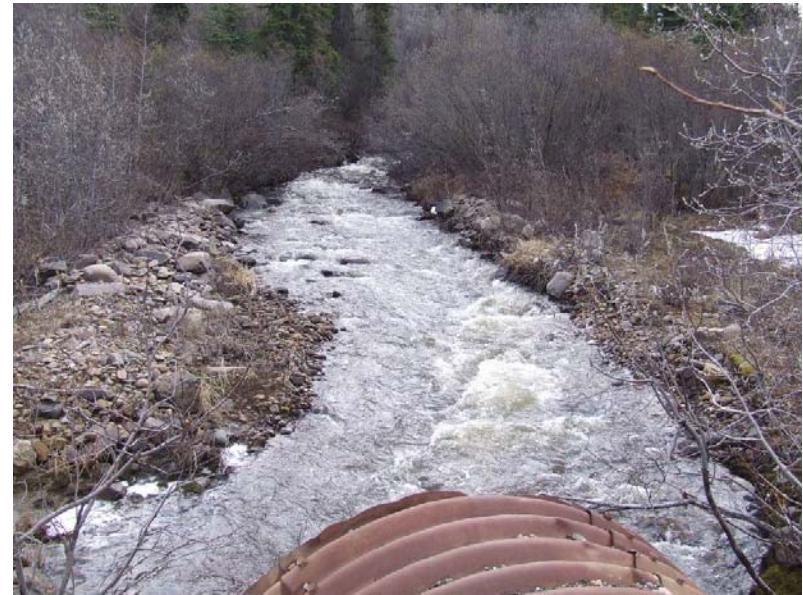
GCULV, looking upstream from mine access road, May 29/12.
