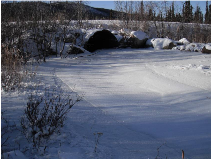
Photo #11; GCULV looking downstream to culvert, Oct 24 th , 2012.
