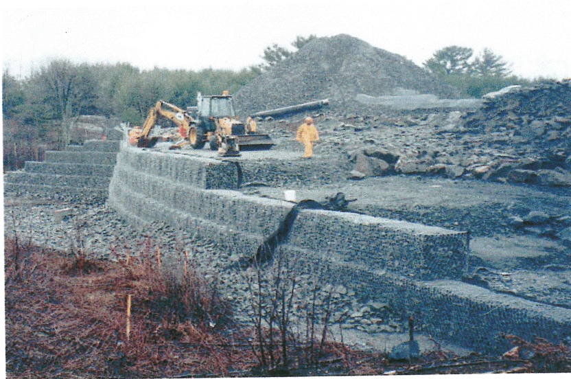
Photograph 1: Gabion Structures - Example
