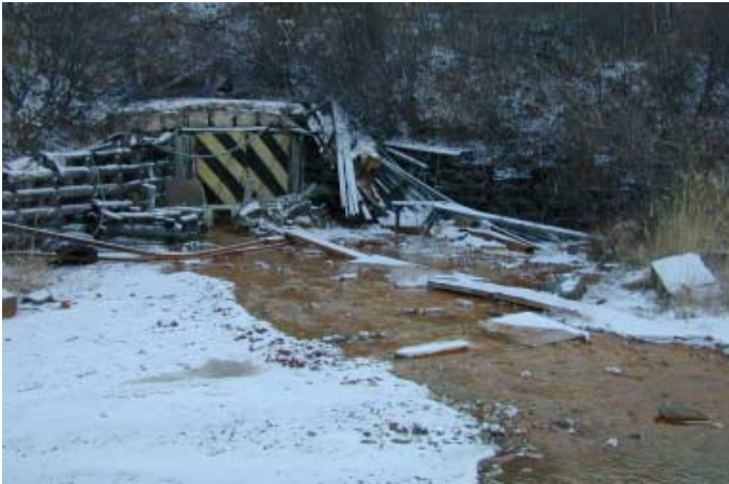
Figure 6 – Galkeno 300 adit discharge, surface flow pattern at the adit.
