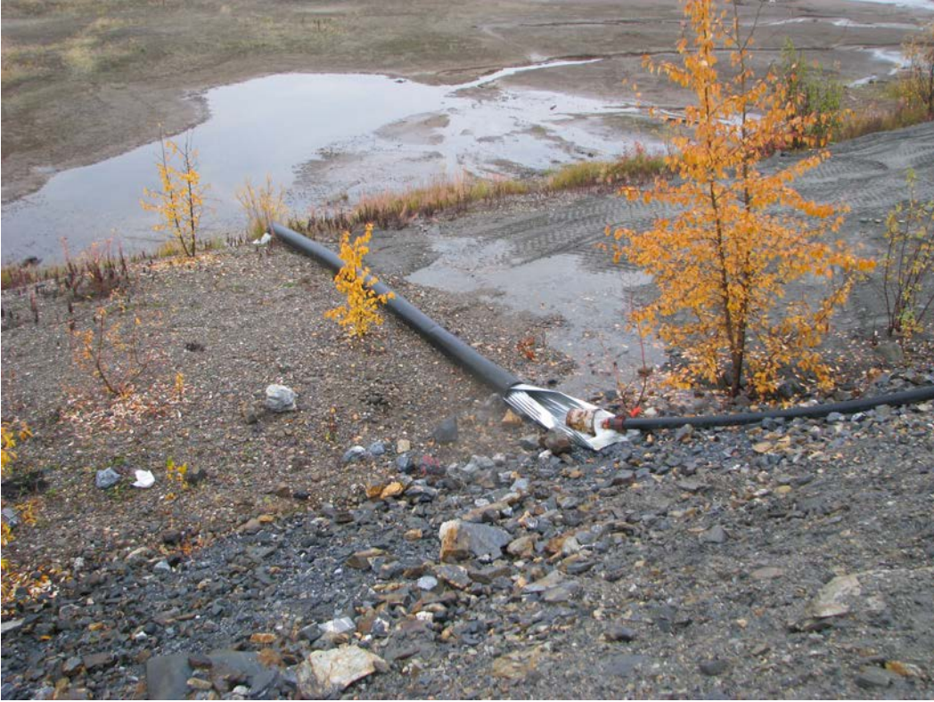
Siphon hose on dam 1 discharging into pond two
