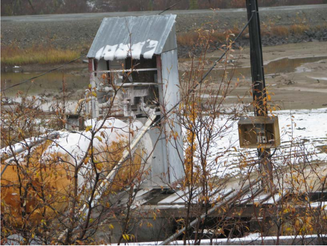
Treatment system from dam 1. Not in use
