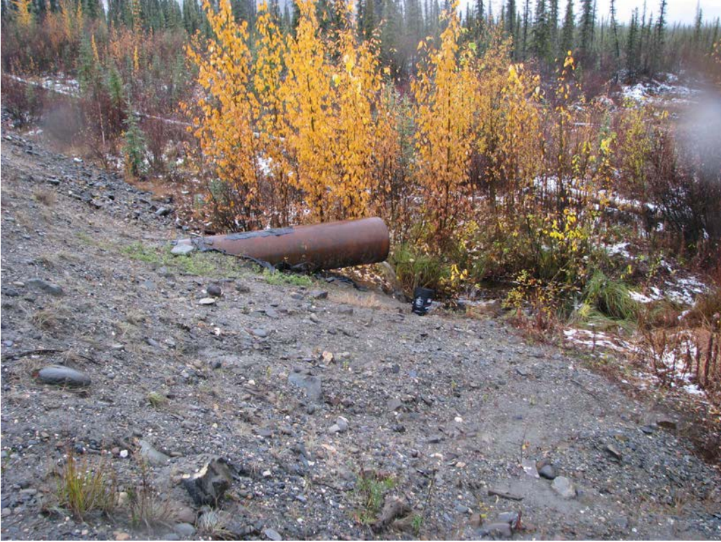
Outlet pipe on dam three. Some flow
