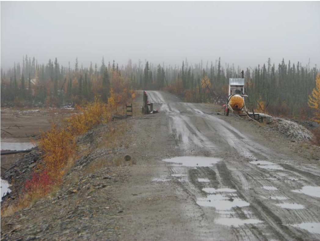
Water treatment system on dam 2 at location of low level structure
