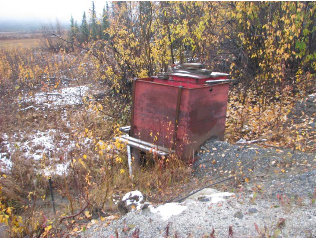
Decant system from dam 1. Water level well below decant invert.
