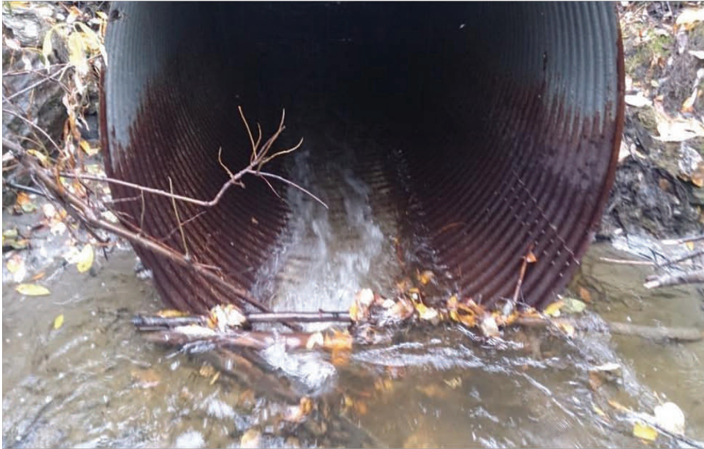
Photo 7: Site R4—Eagle Creek upstream of the culvert (downstream).
