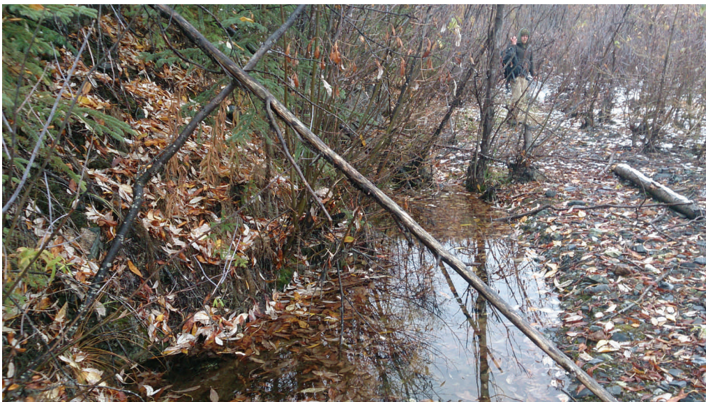
Photo 34: Site GWCC-3—Seepage from rock dump into side channel.
