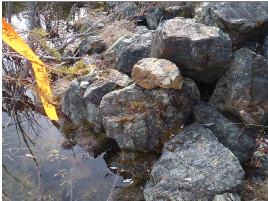
Photo 18: View of groundwater seepage Site GWCC-2. Photo taken on September 21, 2014.
