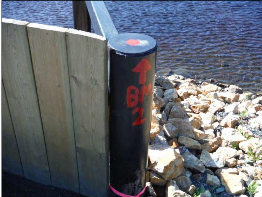
Benchmark 2. Top of steel abutment at outlet of Hudgeon Lake (north side)
